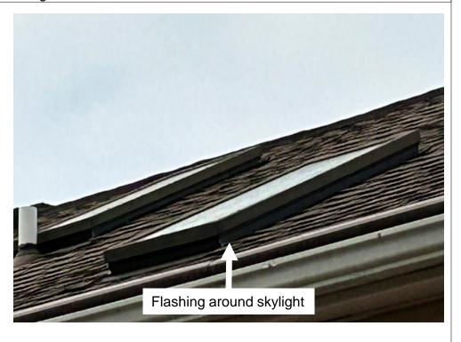
Item 2 Roof to Skylight Flashing – Flashing to protect sides of skylight to prevent against combustible debris ignition and embers.
