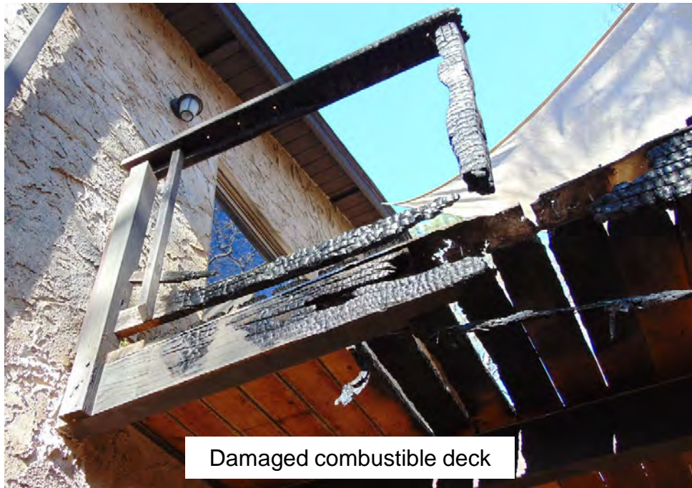
Damaged combustible deck
