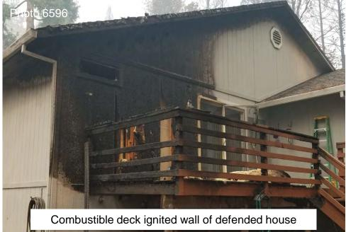
Item 29 Deck-to-Wall Intersection – Providing a 2 ft high noncombustible barrier up from deck along house exterior can reduce ignition.
