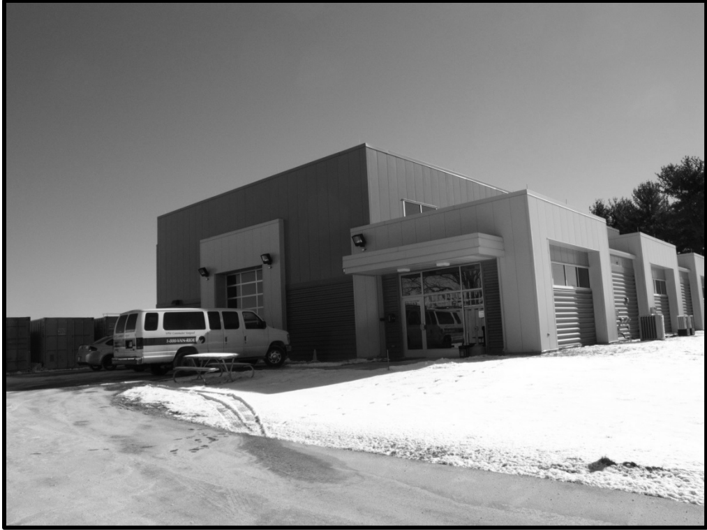
M_20_47_2015_01_28_013. Building 207, north and west elevations
