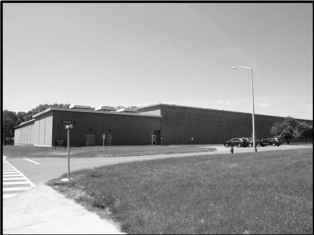
M_20_47_2015_05_14_036. Building 302, north elevation
