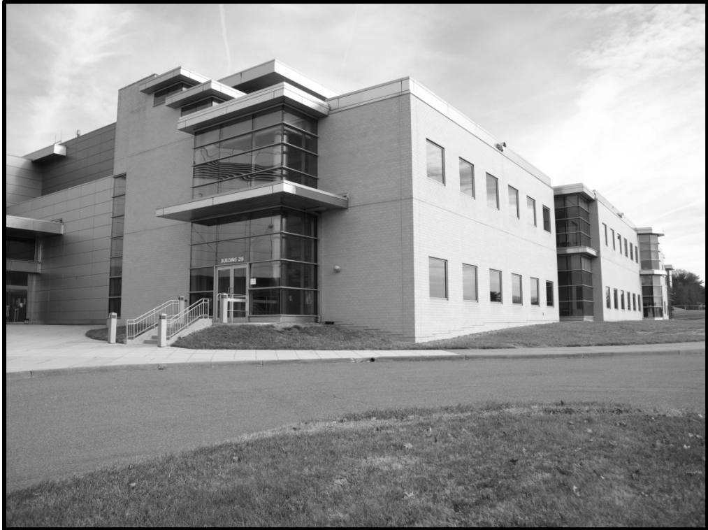
M_20_47_2014_12_04_016. Building 216, west and south elevations
