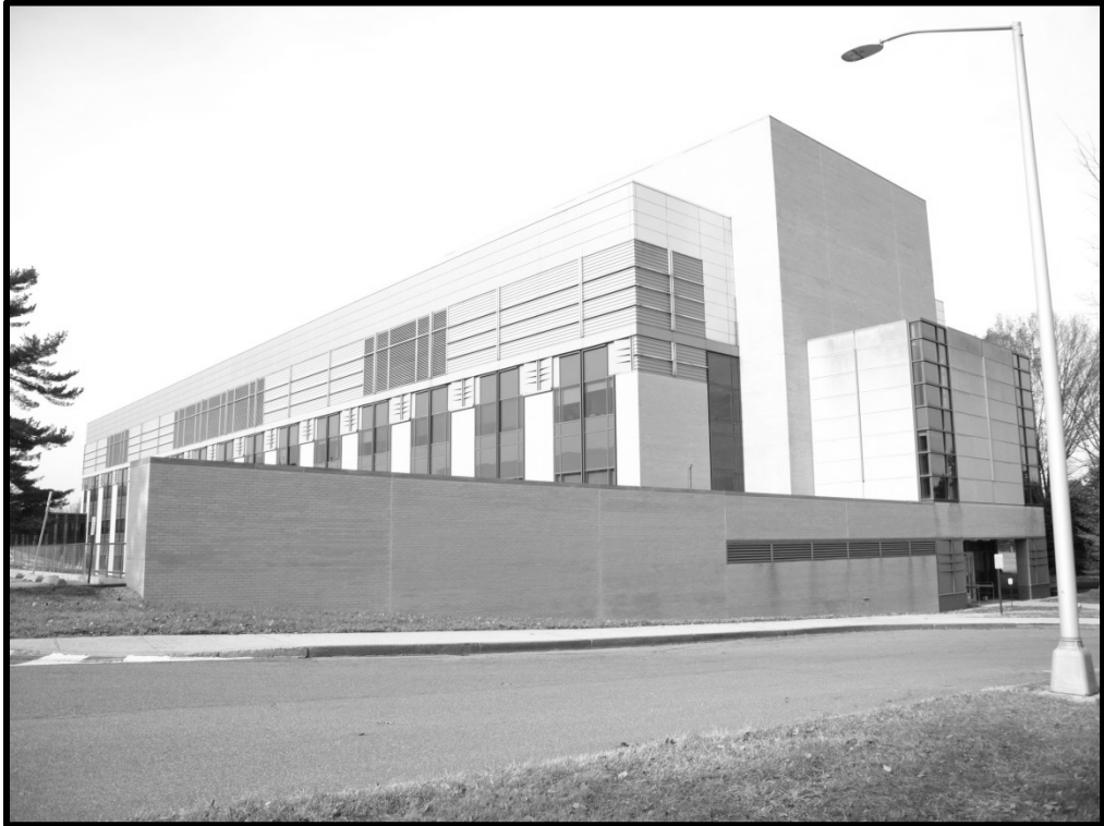
M_20_47_2014_12_04_008. Building 227, east and south elevations
