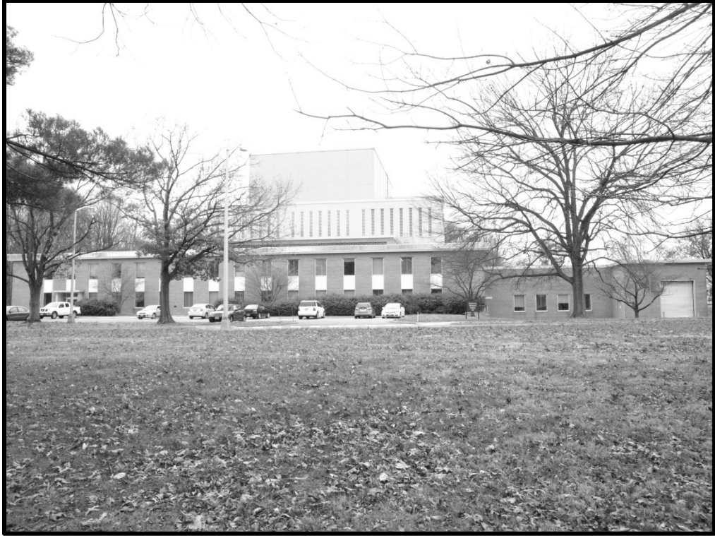
M_20_47_2014_12_04_009. Building 202, east elevation
