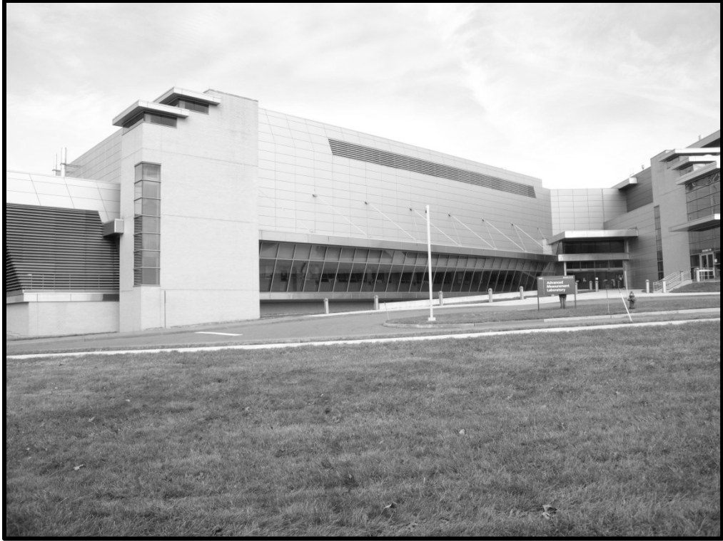
M_20_47_2014_12_04_015. Building 215, northwest elevation
