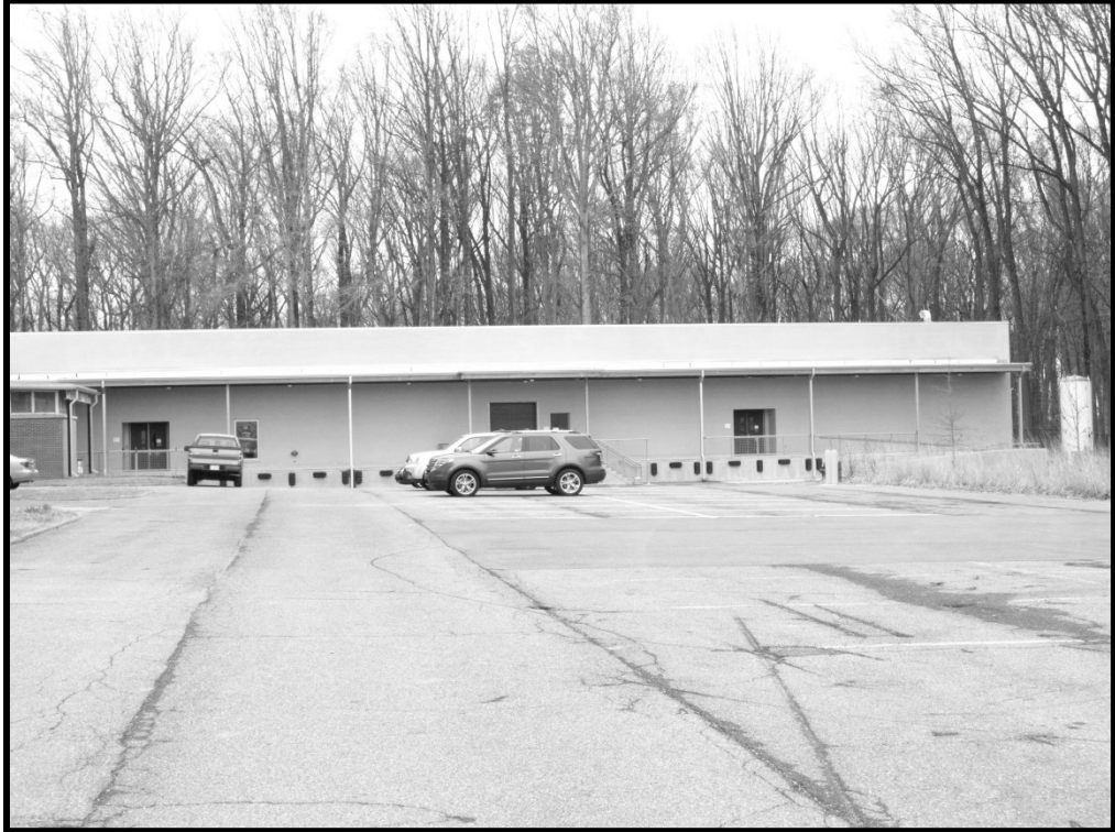
M_20_47_2014_12_04_010. Building 203, north elevation
