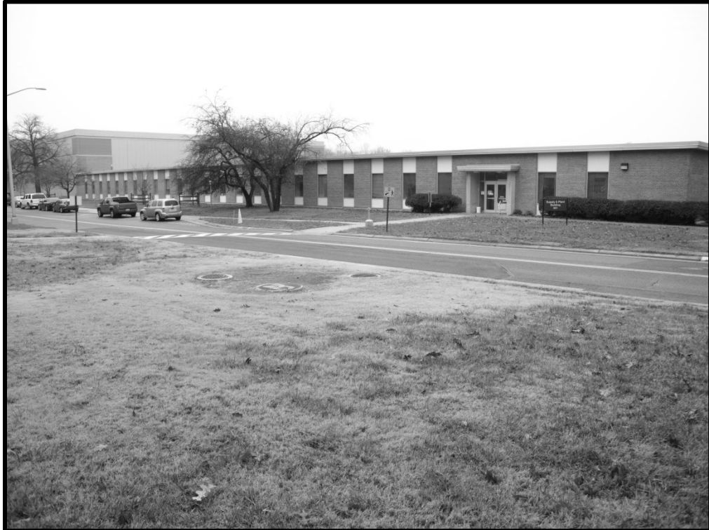
M_20_47_2014_12_03_030. Building 301, east elevation
