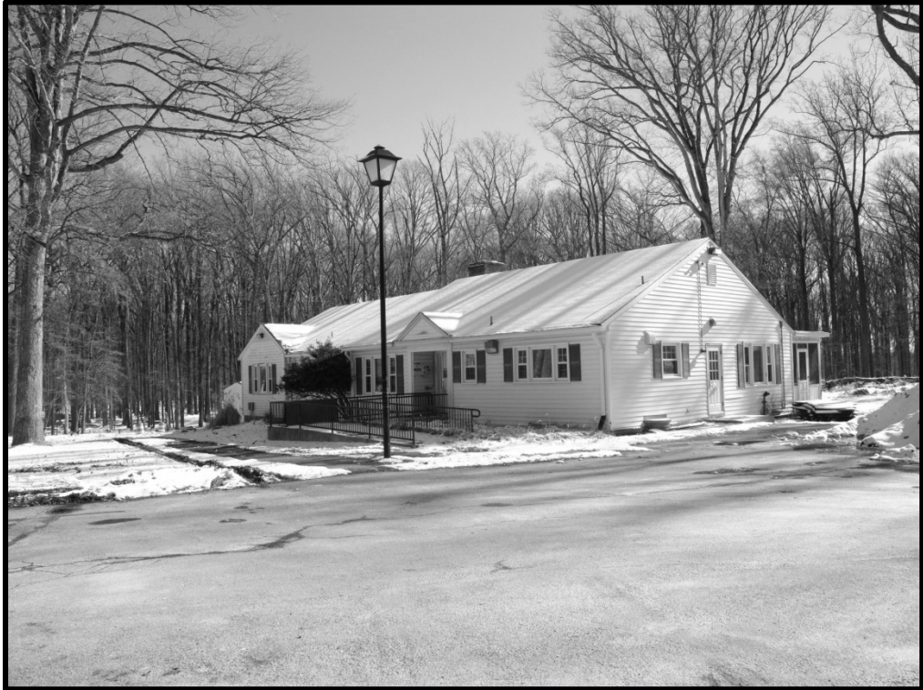
M_20_47_2015_01_28_044. Building 308, north elevation
