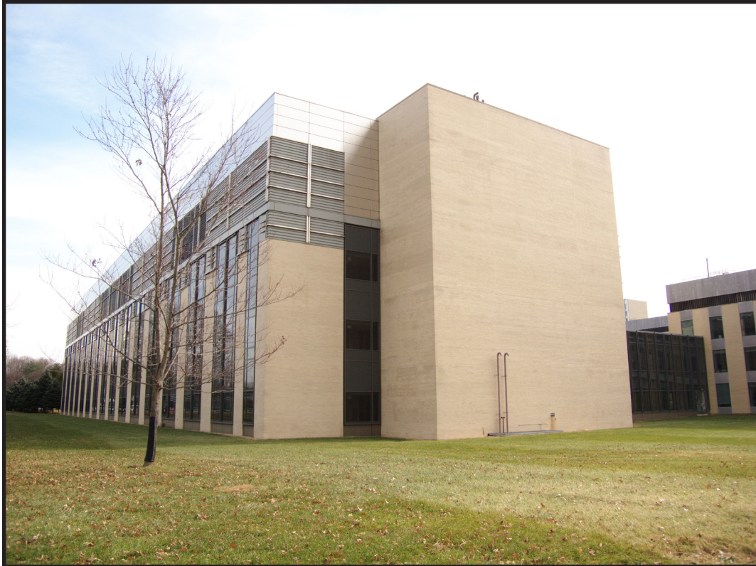
Figure 7.15 Building 227, North and West Elevations (Source: RCG&A 2014).
