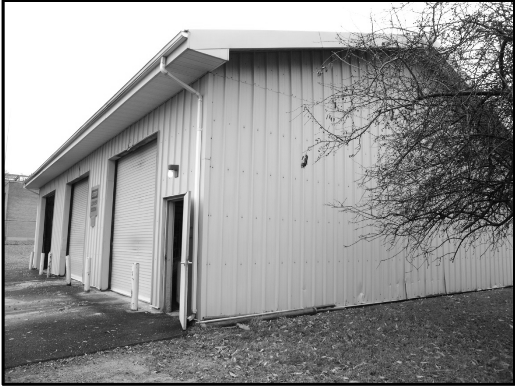
M_20_47_2014_12_03_043. Building 311, north and east elevations
