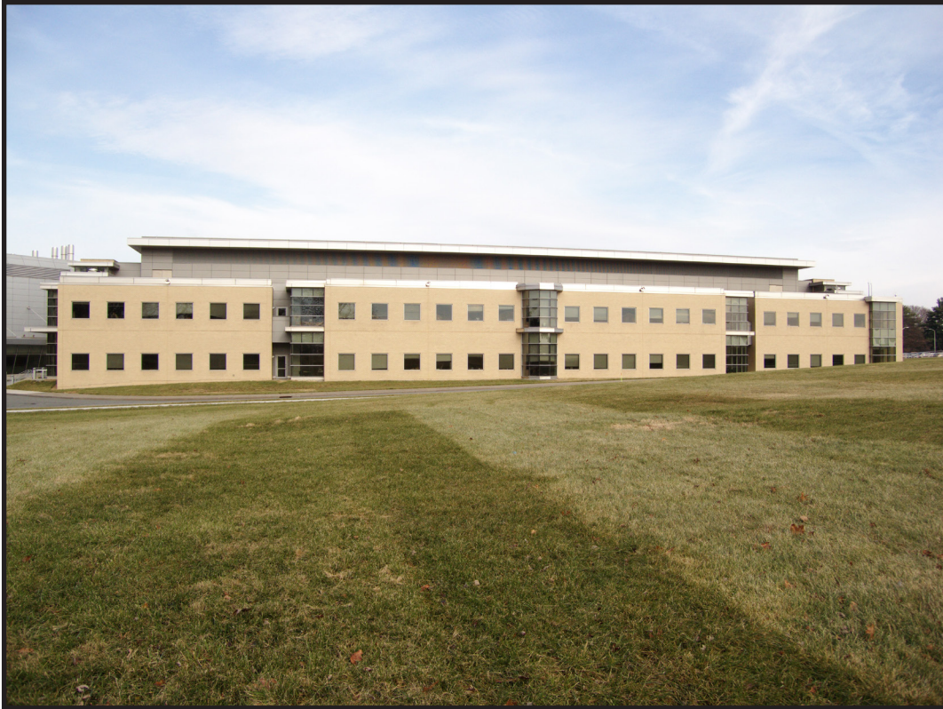
Figure 7.21 Building 216, South Elevation (Source: RCG&A 2014).
