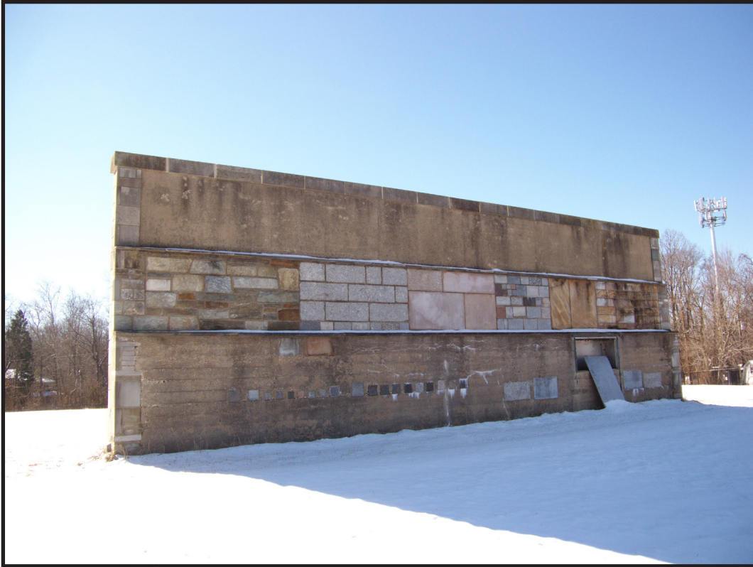
Figure 7.26 Test Wall, North Elevation (Source: RCG&A 2015).
