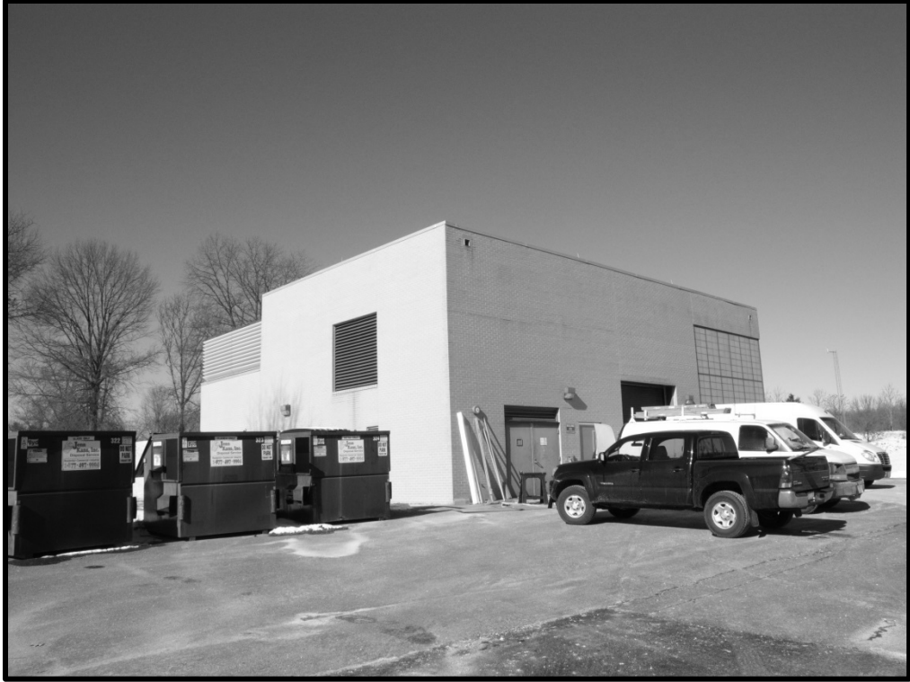
M_20_47_2015_01_28_035. Building 312, east and south elevations
