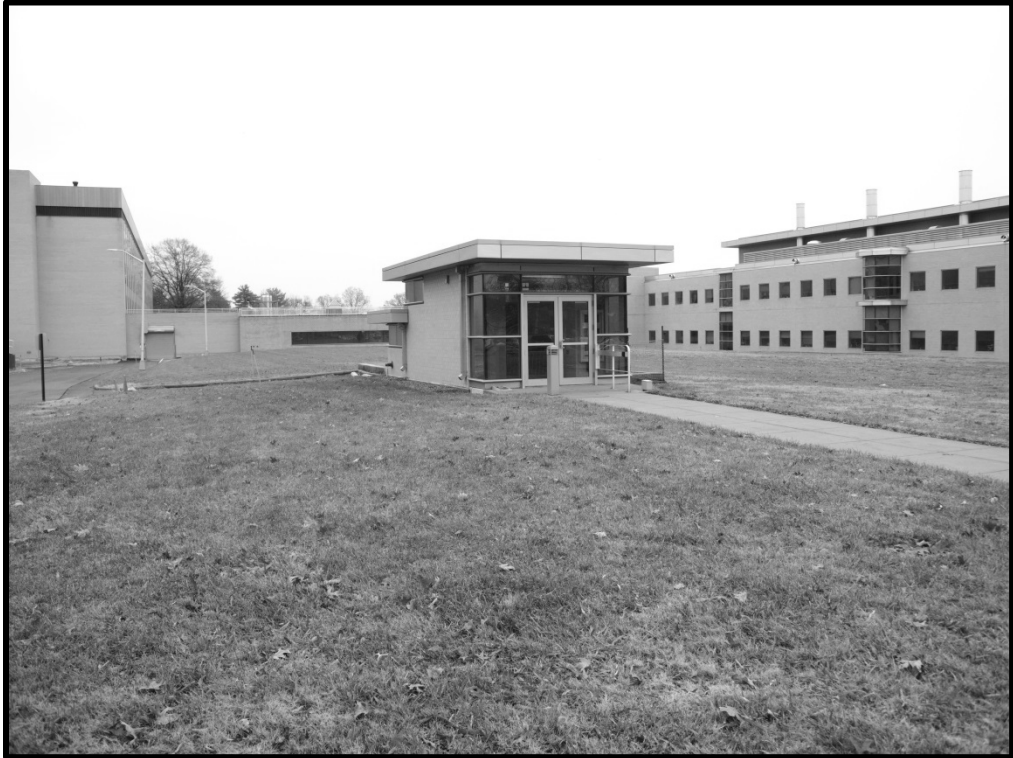
M_20_47_2014_12_04_018. Building 219, looking east
