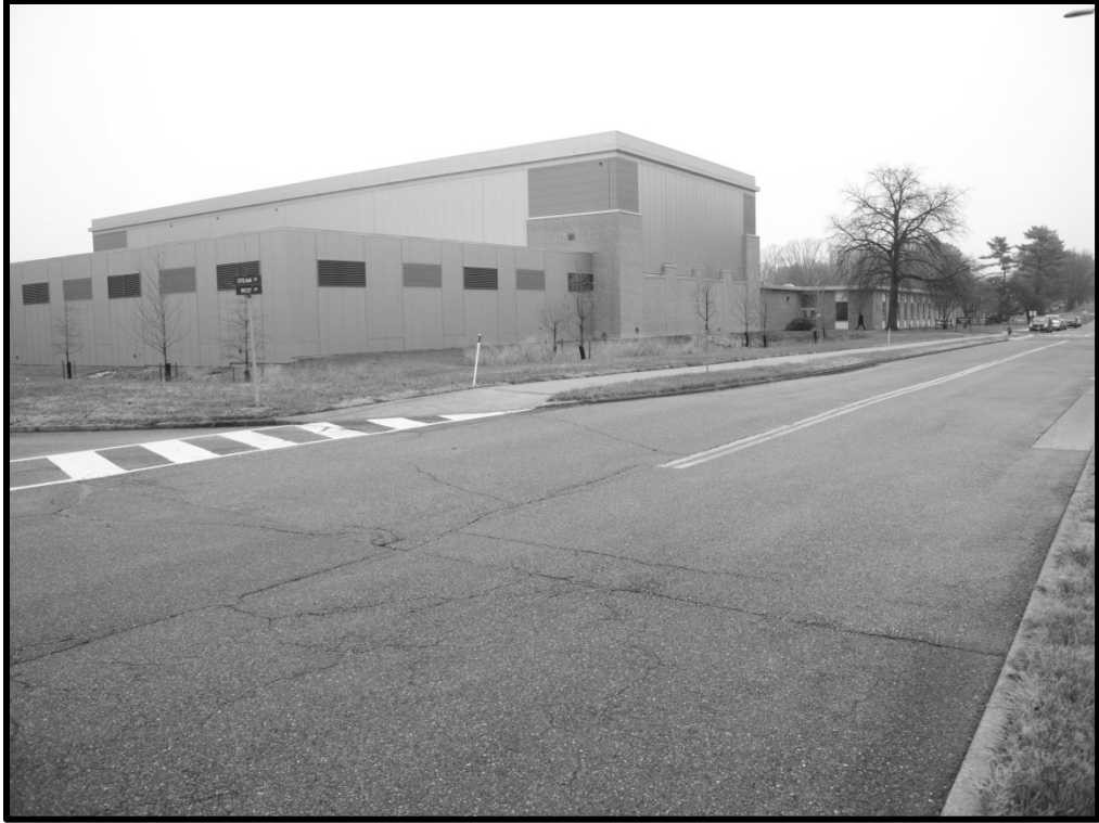
M_20_47_2014_12_03_031. Building 301, south and east elevations
