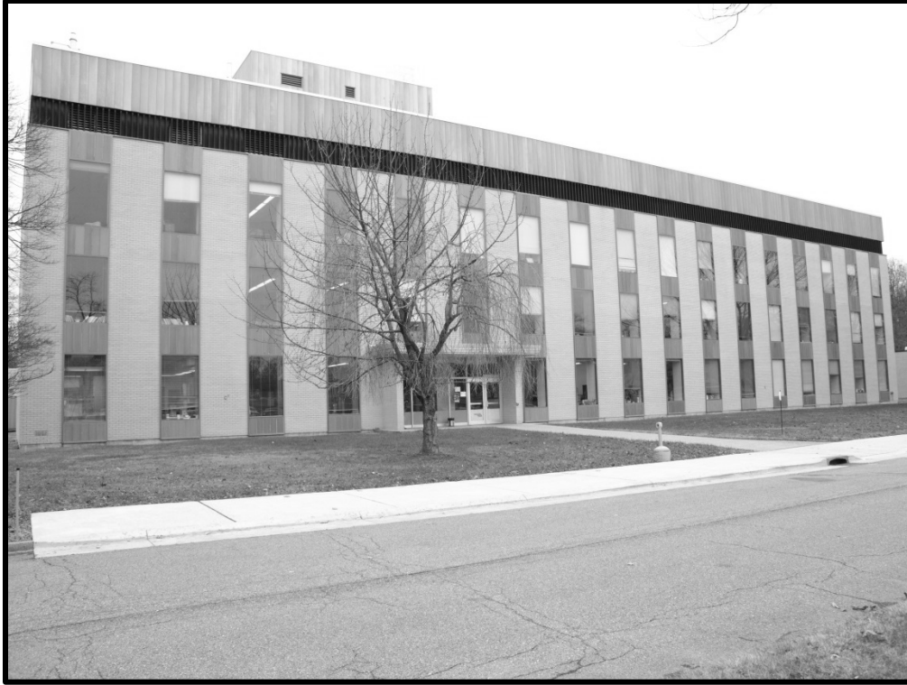
M_20_47_2014_12_04_025. Building 245, north elevation
