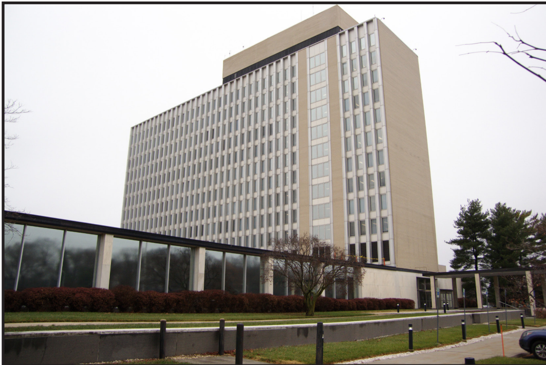
Figure 7.19 Administration Building (Source: RCG&A 2014)
