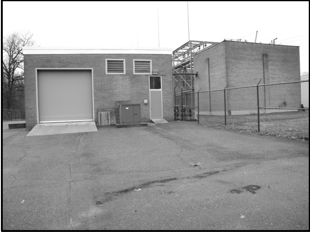
M_20_47_2014_12_03_039. Building 306, north elevation
