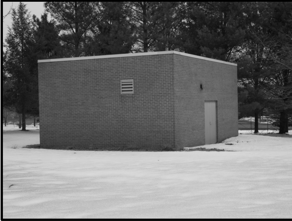
M_20_47_2015_03_03_041. Building 315, east and south elevations
