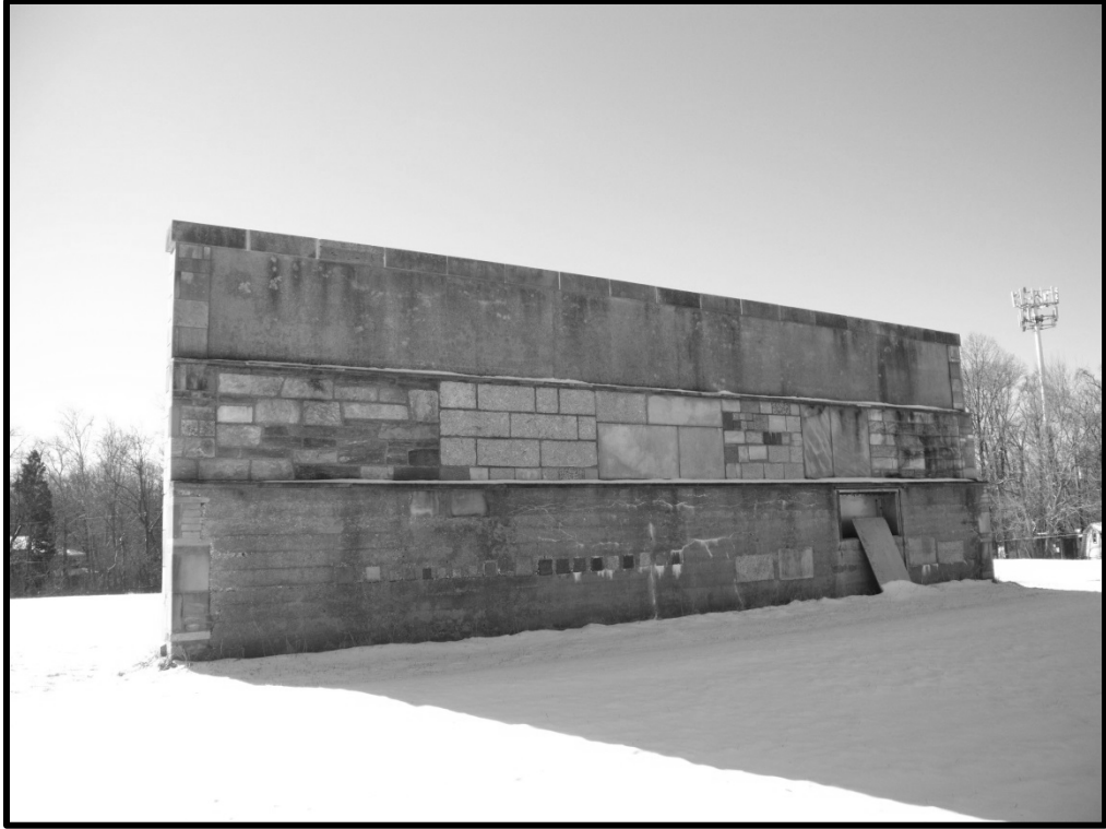
M_20_47_2015_01_28_047. Masonry test wall, looking south
