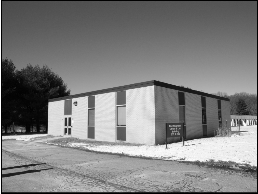
M_20_47_2015_01_28_023. Building 237, south and east elevations
