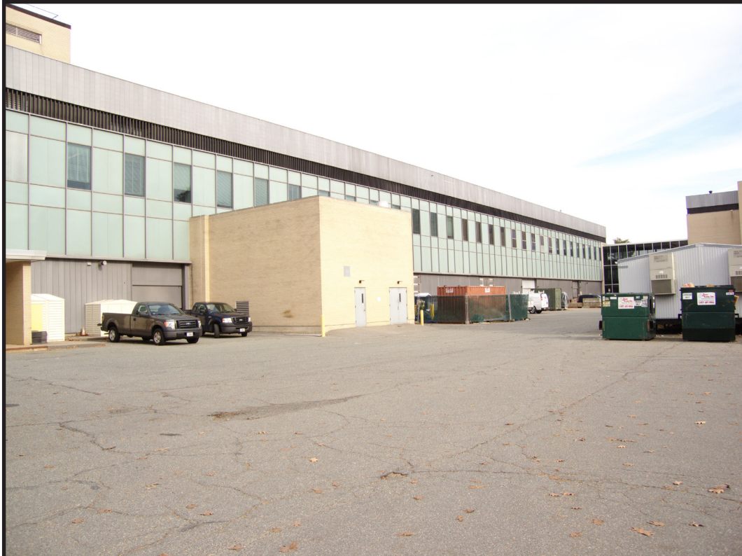
Figure 7.9 Building 226, South Elevation (Source: RCG&A 2014).
