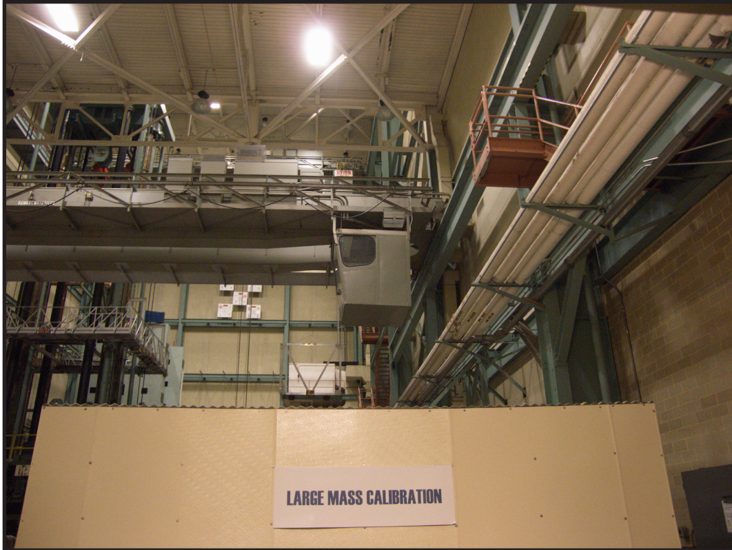
Figure 7.25 Highbay, Building 202 (Source: RCG&A 2015).
