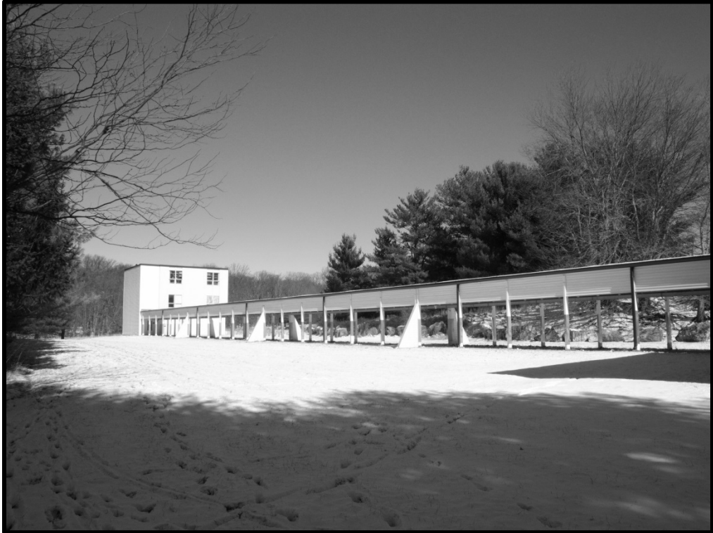
M_20_47_2015_01_28_024. Building 238, south and west elevations
