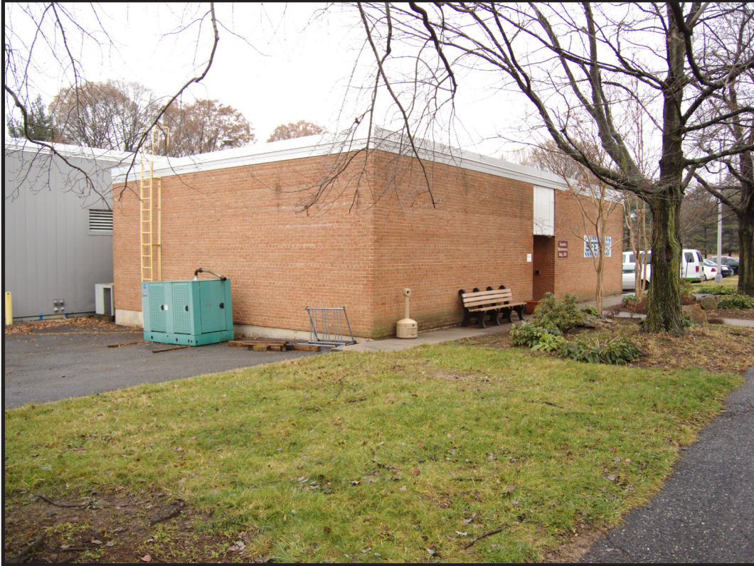
Figure 7.29 Building 309, East Elevation (Source: RCG&A 2014).
