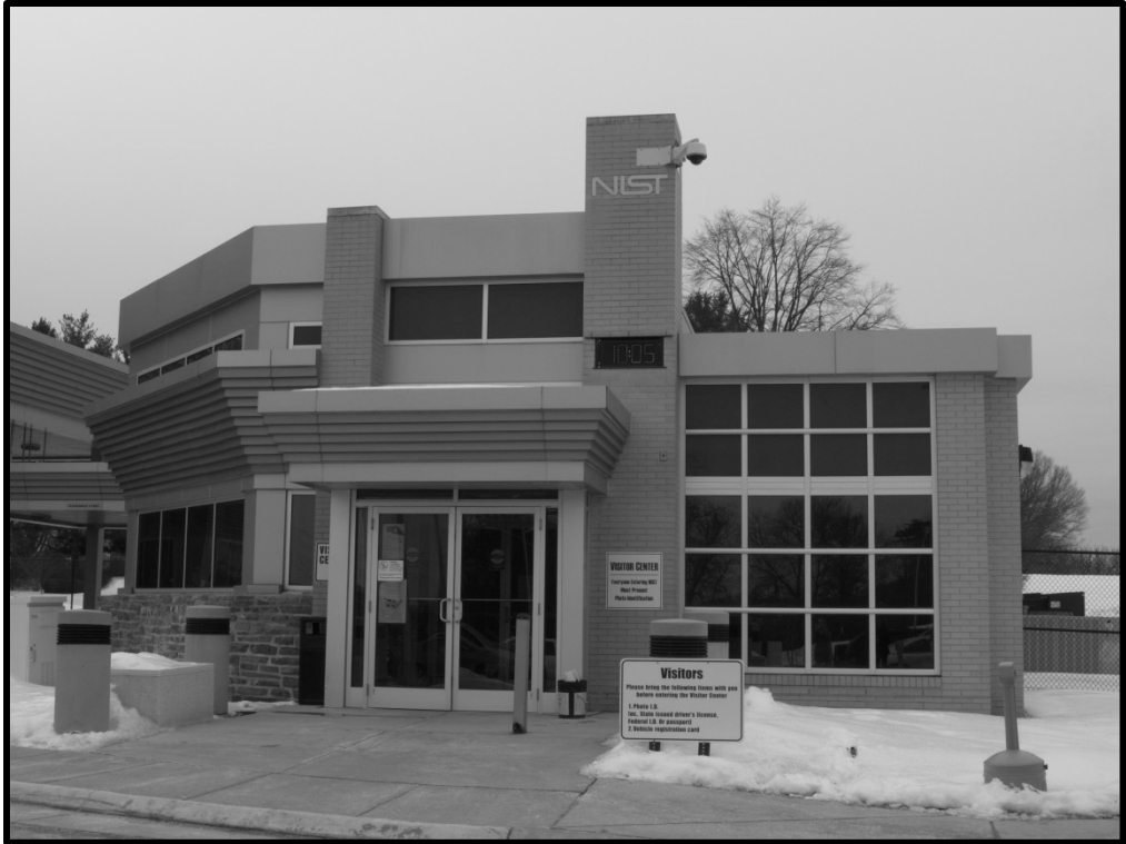
M_20_47_2015_03_03_027. Building 103, north elevation
