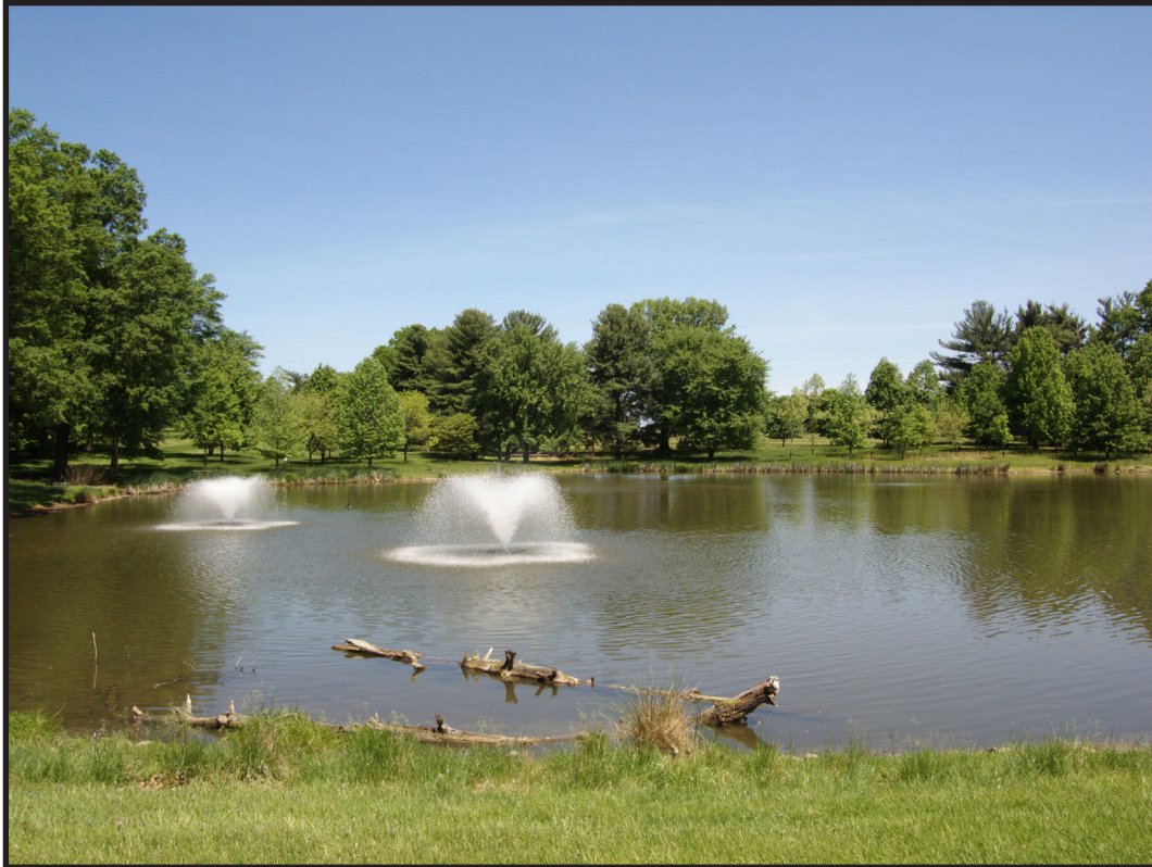
Figure 7.40 Stormwater Management Pond 1, Looking North (Source: RCG&A 2014).
