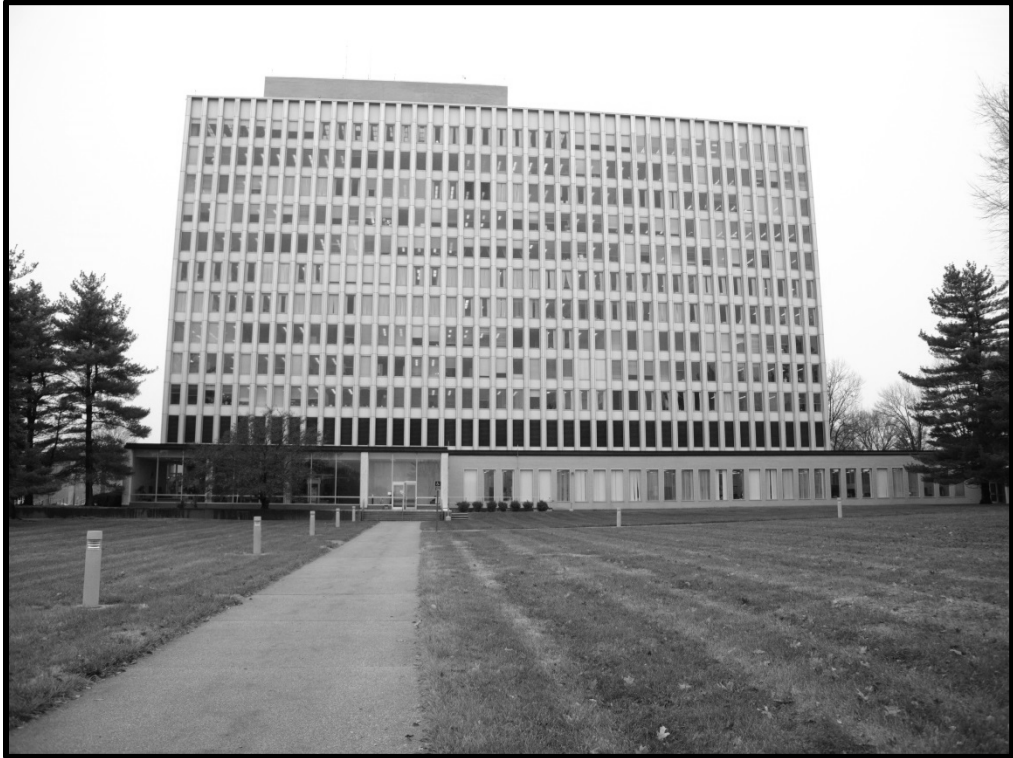
M_20_47_2014_12_03_002. Building 101, north elevation
