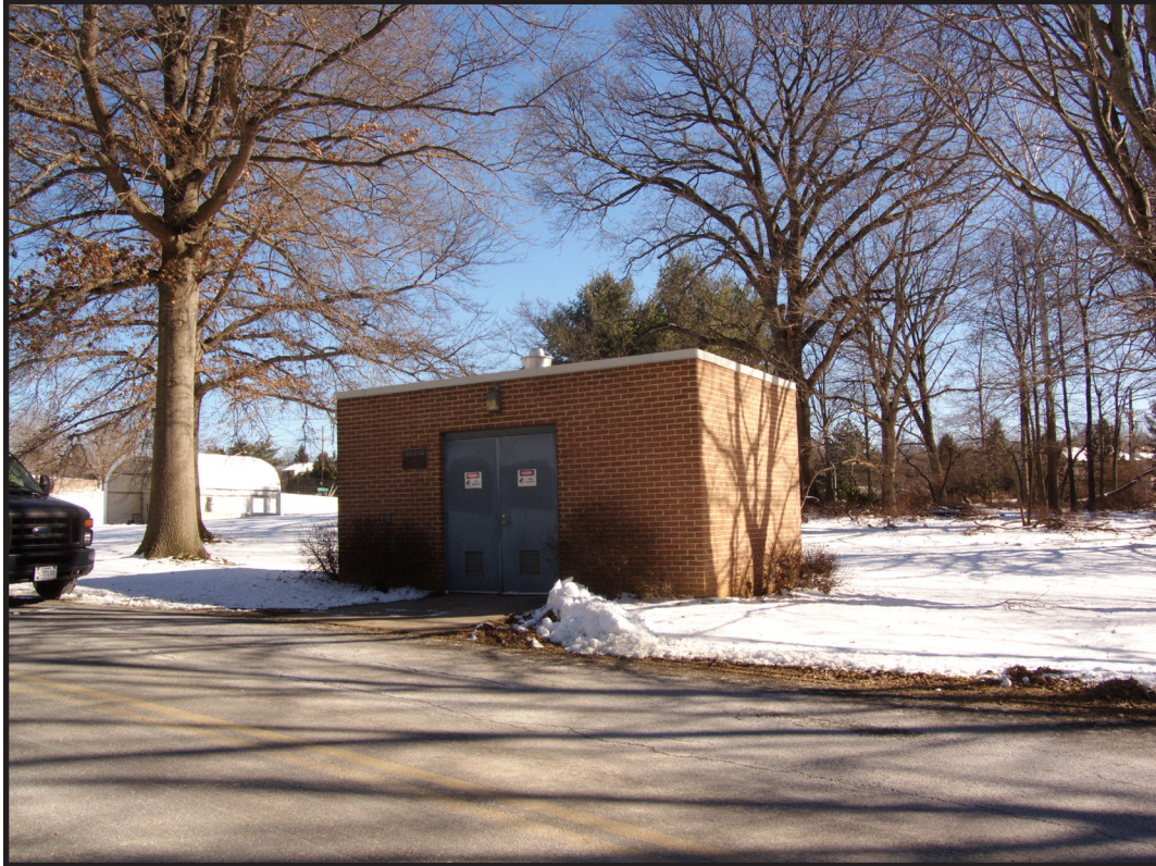
Figure 7.30 Building 313, West and South Elevations (Source: RCG&A 2014).
