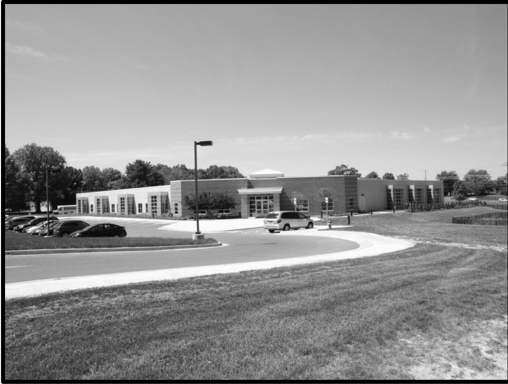
M_20_47_2015_05_14_029. Building 320, looking southwest
