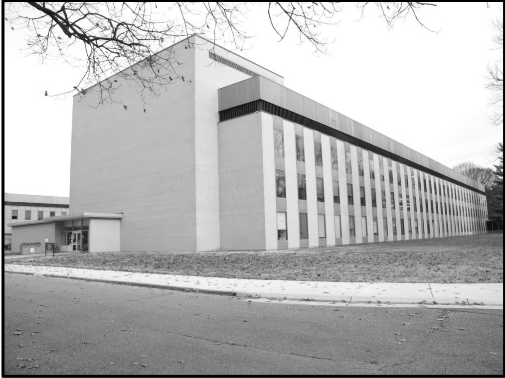
M_20_47_2014_12_04_007. Building 224, west and south elevations
