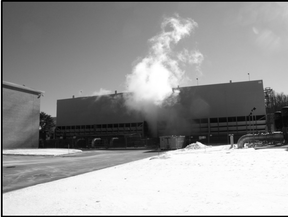
M_20_47_2015_01_28_037. Building 305, north elevation
