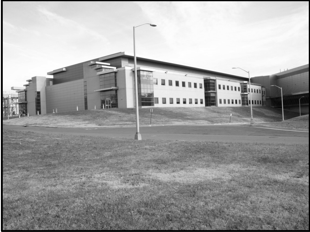
M_20_47_2014_12_04_017. Building 217, east and south elevations
