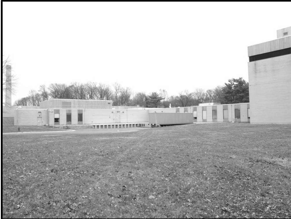
M_20_47_2014_12_04_026. Building 245, looking southwest
