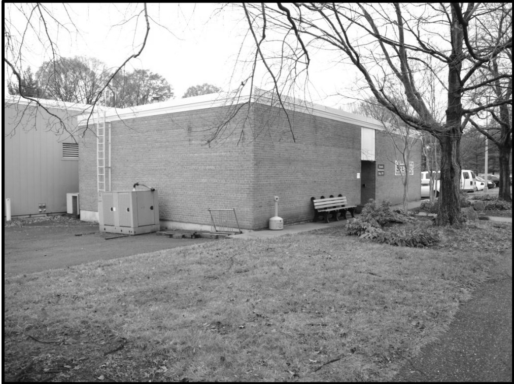
M_20_47_2014_12_03_034. Building 309, east elevation
