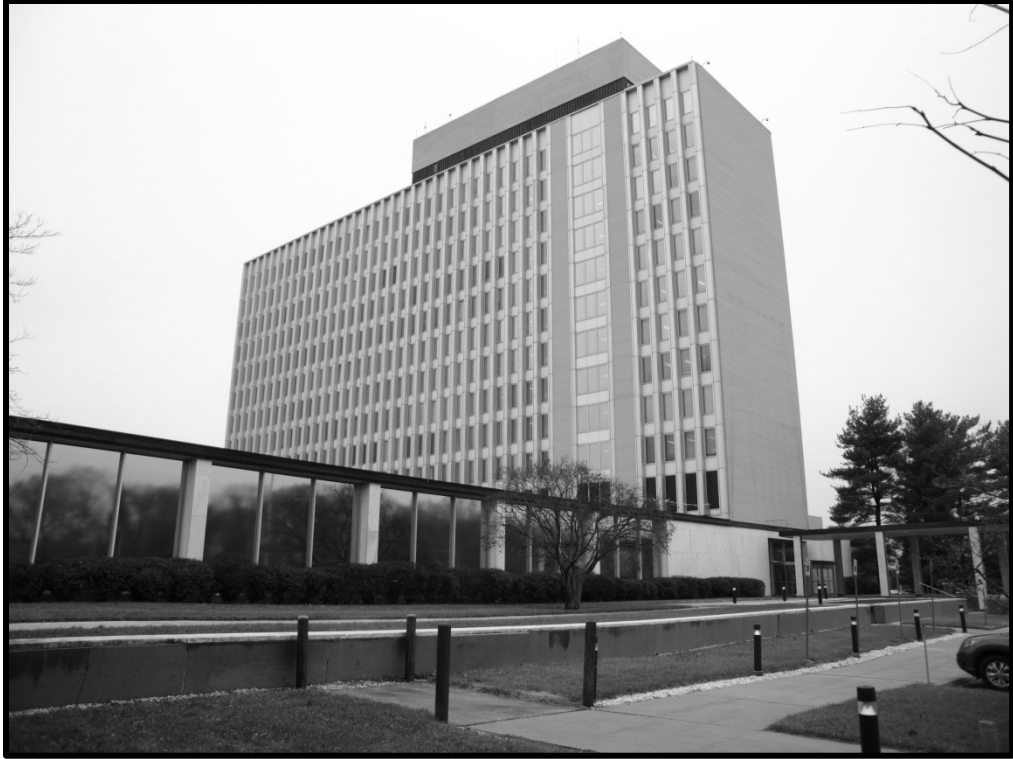
M_20_47_2014_12_03_001. Building 101, looking northwest
