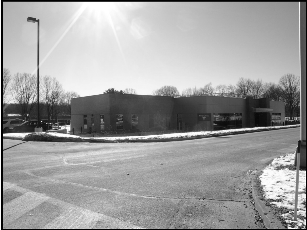
M_20_47_2015_03_03_028. Building 318, north and east elevations
