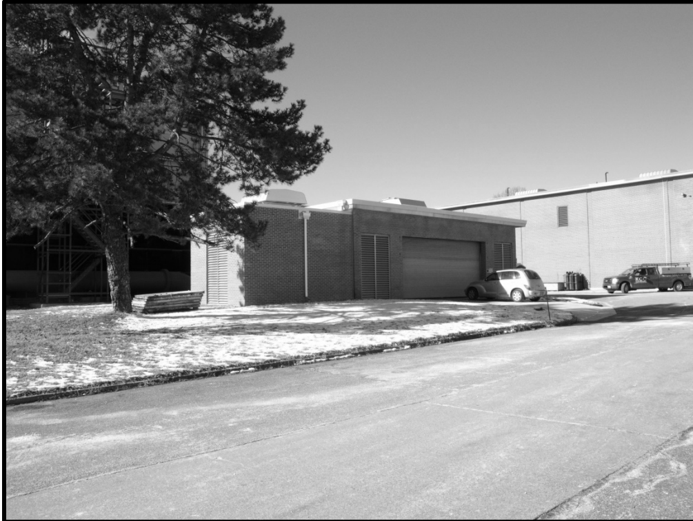
M_20_47_2015_01_28_038. Building 316, south and east elevations
