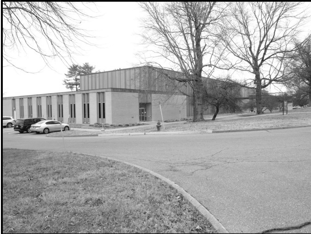
M_20_47_2014_12_04_020. Building 231, south and east elevations
