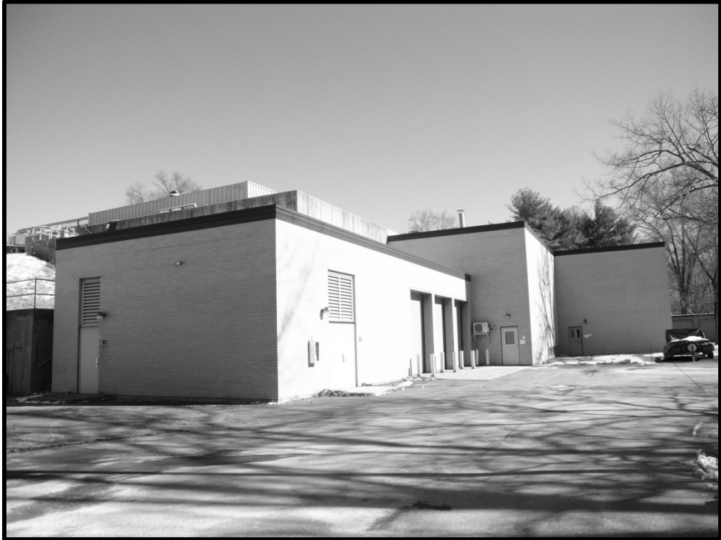
M_20_47_2015_01_28_012. Building 206, west and south elevations
