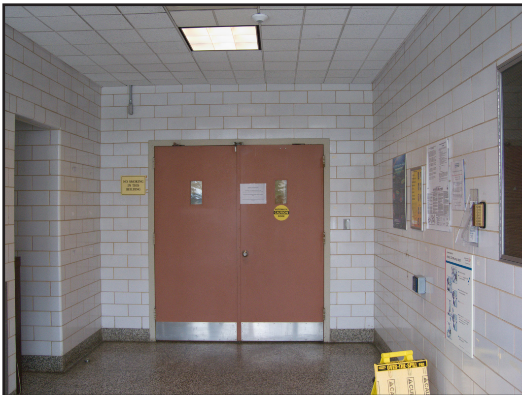
Figure 7.23 Interior, Lobby Building 202 (Source: RCG&A 2015).
