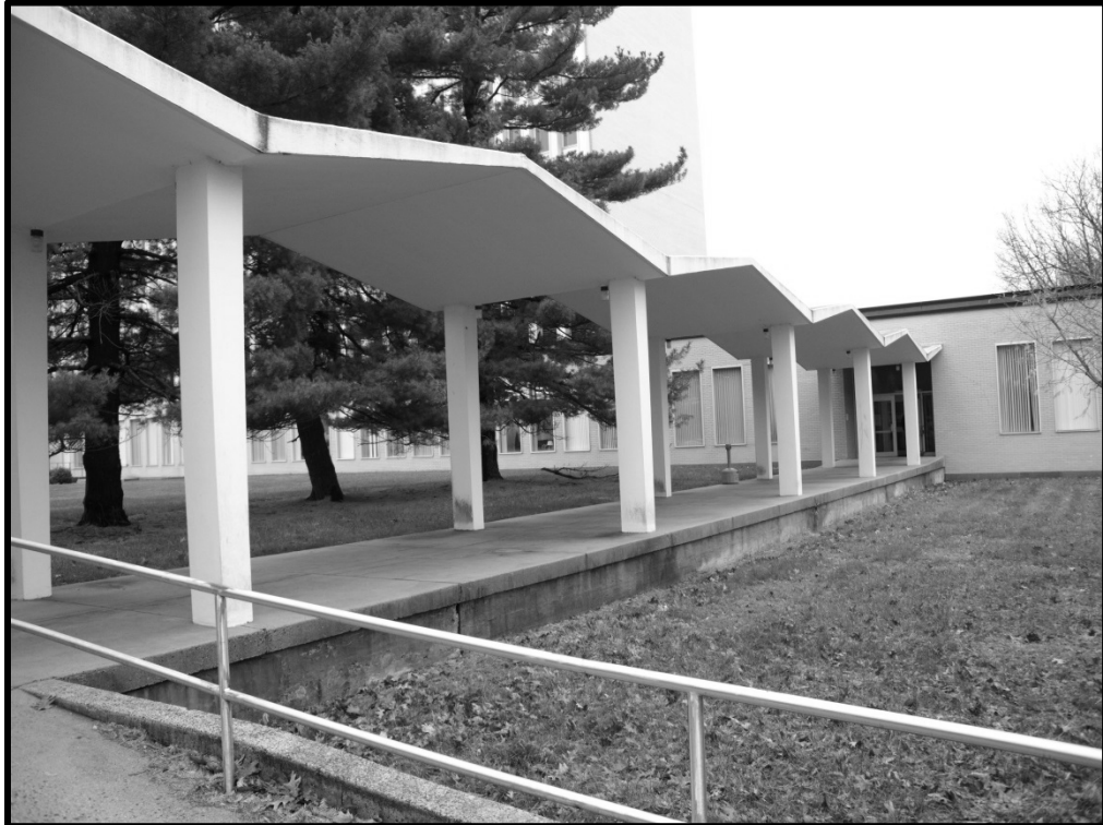
M_20_47_2014_12_03_006. Walkway from Building 101 to Building 225
