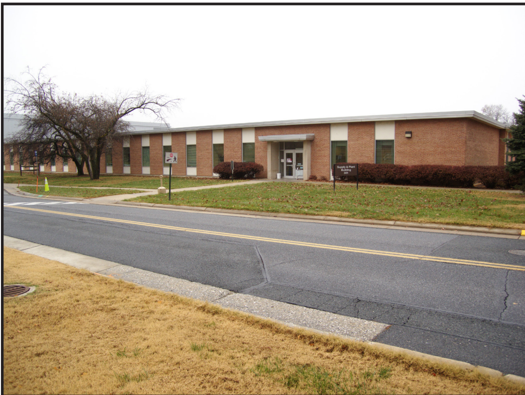
Figure 7.28 Building 301, East Elevation (Source: RCG&A 2014).
