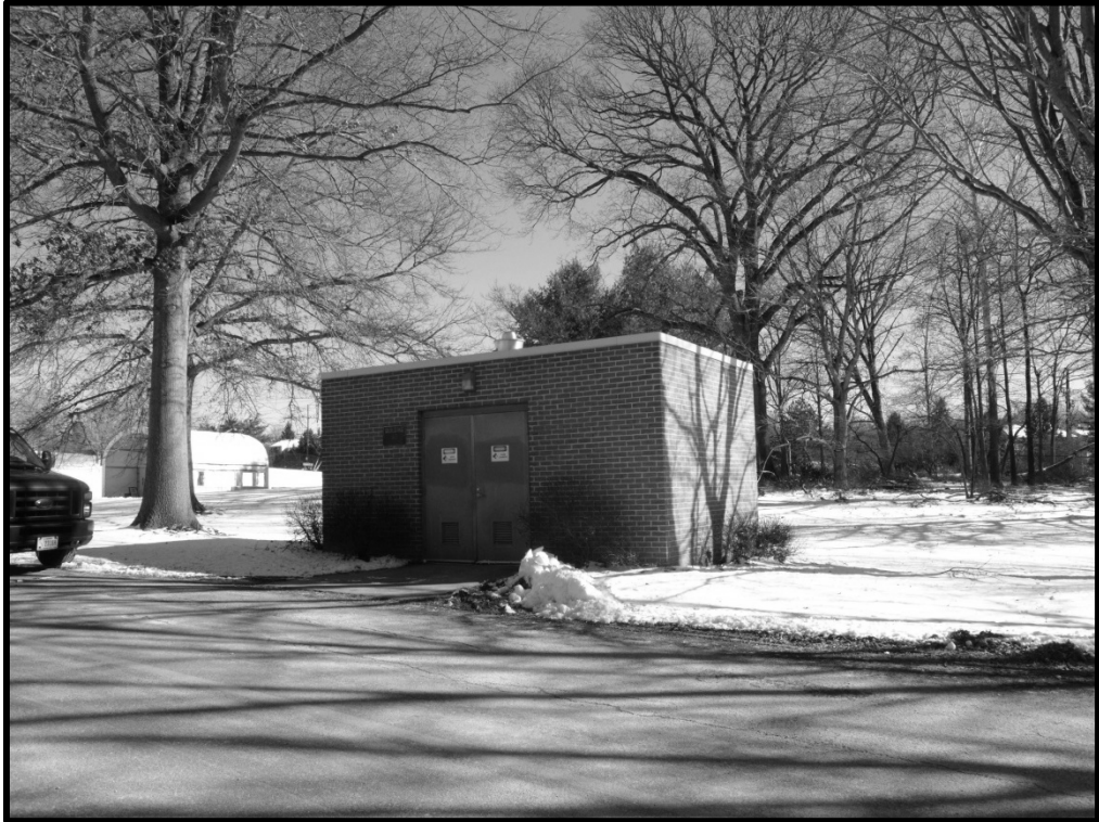
M_20_47_2015_01_28_040. Building 313, west and south elevations
