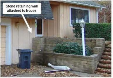
Item 34 Attached Retaining Walls - Replace retaining wall length equal to two times retaining wall height with noncombustible components.
