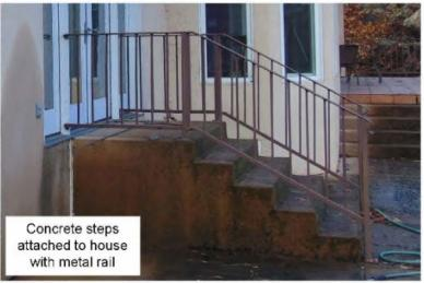
Item 32 Stairs Connected to Residence – Use a noncombustible material for exterior stairs attached to noncombustible barrier/section between steps and house and between handrails and house (min 1') or replace with noncombustible handrail.
