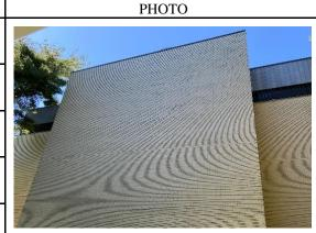
Beige face brick (Gray PBS No. 36.797) extends along the entire windowless east elevation. The use of brick cladding on the first three floors of the building identifies these as occupied floors, whereas the aluminum banding above it indicates mechanical and utility spaces. The third floor is capped with an extruded aluminum cornice with an Alcoa #2020 Grey finish and the base consists of cement stucco parging.
