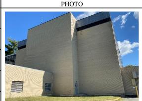
Beige face brick (Gray PBS No. 36.797) extends along the entire windowless west elevation. The use of brick cladding on the first three floors of the building identifies these as occupied floors, whereas the aluminum banding above it indicates mechanical and utility spaces. The third floor is capped with an extruded aluminum cornice with an Alcoa #2020 Grey finish and the base consists of cement stucco parging.
