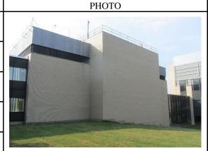
Beige face brick (Gray PBS No. 36.797) extends along the entire windowless east elevation. The use of brick cladding on the first three floors of the building identifies these as occupied floors, whereas the aluminum banding above it indicates mechanical and utility spaces. The third floor is capped with an extruded aluminum cornice with an Alcoa #2020 Grey finish and the base consists of cast-in-place concrete.
