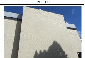
Beige face brick (Gray PBS No. 36.797) extends along the entire windowless east elevation. The use of brick cladding on the first three floors of the building identifies these as occupied floors, whereas the aluminum banding above it indicates mechanical and utility spaces. The third floor is capped with an extruded aluminum cornice with an Alcoa #2020 Grey finish and the base consists of cement stucco parging.
