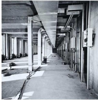
A14: Construction of the second type of ventilation system installed in the lab spaces connected to the corridors. (Source: NIST)
