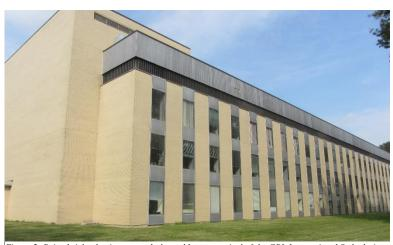
Figure 2: Beige brick, aluminum spandrels, and louvers typical of the GPL International Style design. (Image: MTFA 2021)
