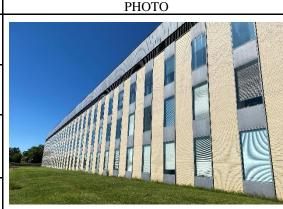
The primary cladding of the south exterior elevation is beige face brick (Gray PBS No. 36.797) alternating between bands of plate glass and insulated aluminum window assemblies. The use of brick cladding on the first three floors of the building identifies these as occupied floors. The third floor is capped with an extruded aluminum cornice with an Alcoa #2020 Grey finish and the base consists of cement stucco parging.
