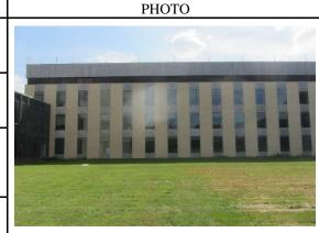
The primary cladding of the north exterior elevation is beige face brick (Gray PBS No. 36.797) alternating between bands of plate glass and insulated aluminum window assemblies. The use of brick cladding on the first three floors of the building identifies these as occupied floors. The third floor is capped with an extruded aluminum cornice with an Alcoa #2020 Grey finish and the base consists of cast-in-place concrete.
