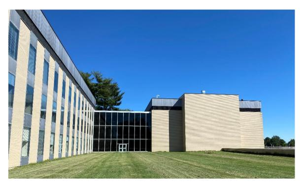
Figure 5: Curtain wall fenestration to the left. Glass concourse contrasts with the fenestration and solid building forms.
