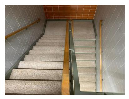
Figure 8: Interior stair hall showing terrazzo, wood handrails, and structural facing tile in different colors.
