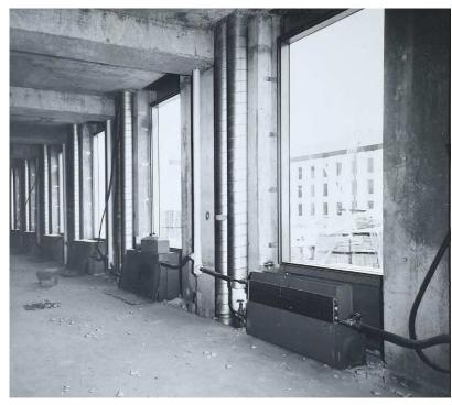
Figure A13: Installation of ventilation and heating/air conditioning. (Source: NIST)
