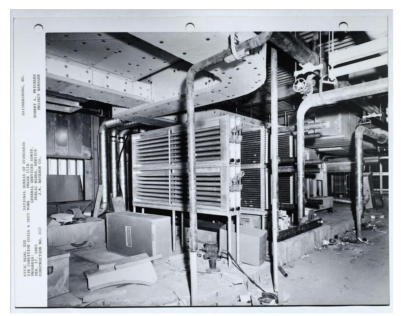
GPL Building 222 Air Condition Coils & Duct Work - February 17, 1965 NIST Library Vertical Files - Gaithersburg Campus. J.W. Bateson Co. Contractors Progress Photos - Phase 111B - Construction 317
