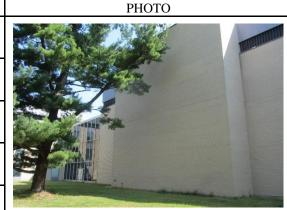
Beige face brick (Gray PBS No. 36.797) extends along the entire windowless west elevation. The use of brick cladding on the first three floors of the building identifies these as occupied floors, whereas the aluminum banding above it indicates mechanical and utility spaces. The third floor is capped with an extruded aluminum cornice with an Alcoa #2020 Grey finish and the base consists of cement stucco parging.
