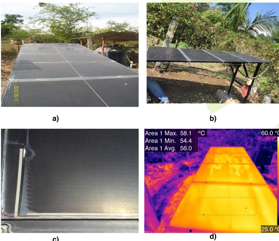
Figure 1. a) Front view of the installation, b) side view of the installation, c) Electro-chemical corrosion, d) Infrared Image
