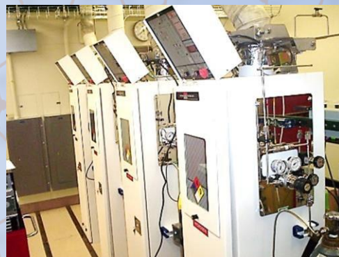
Continuously vented cabinets for hydrogen and methane gas cylinders
