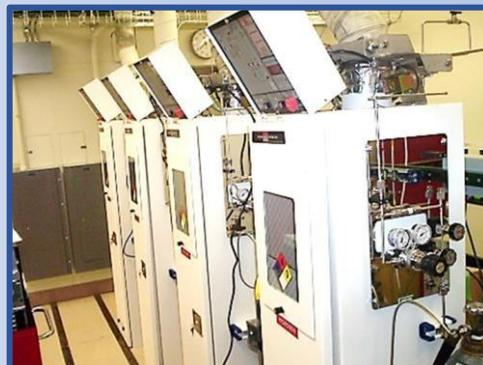
Continuously vented cabinets for hydrogen and methane gas cylinders
