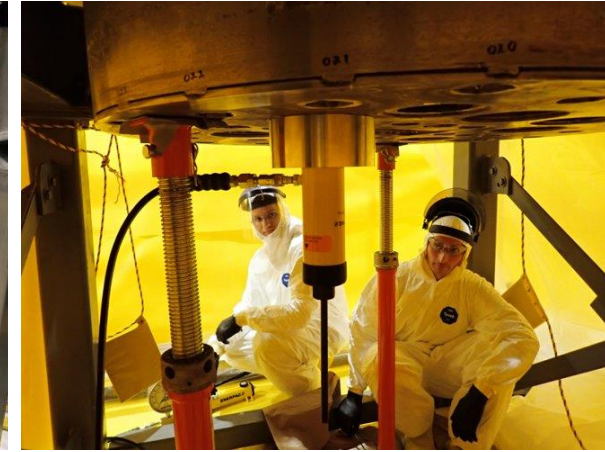
Testing and repair
