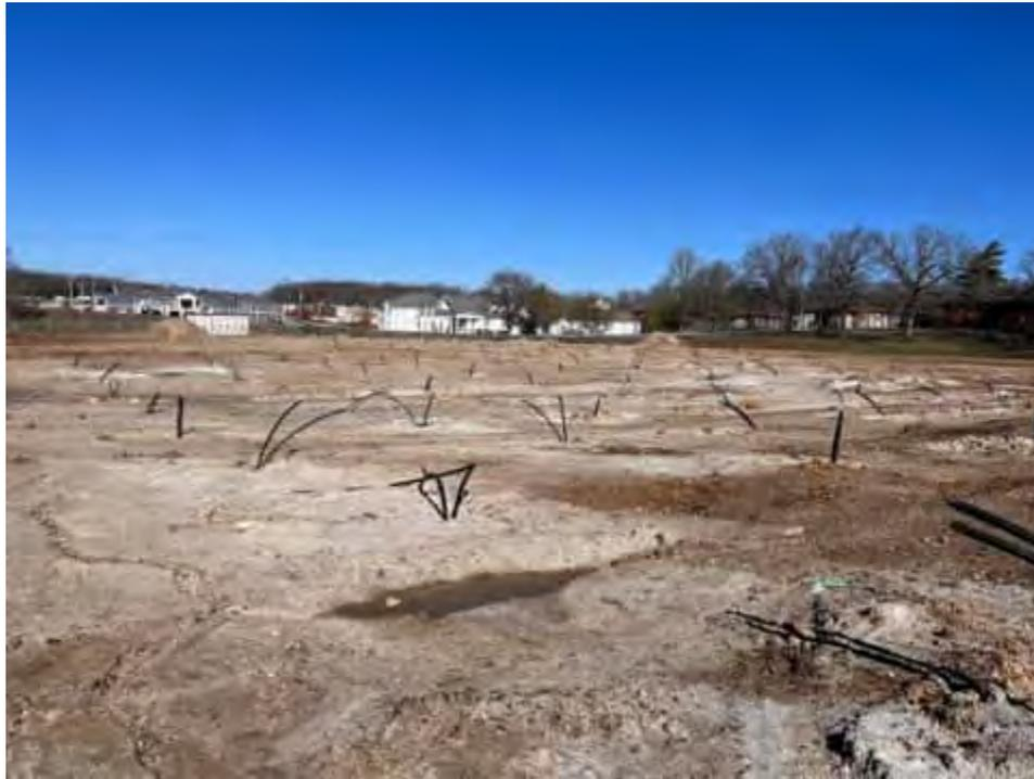
Photograph B-13: Low area of fill in the western portion of the APE with flex piping installed for the geothermal well. Photograph facing Northwest.
