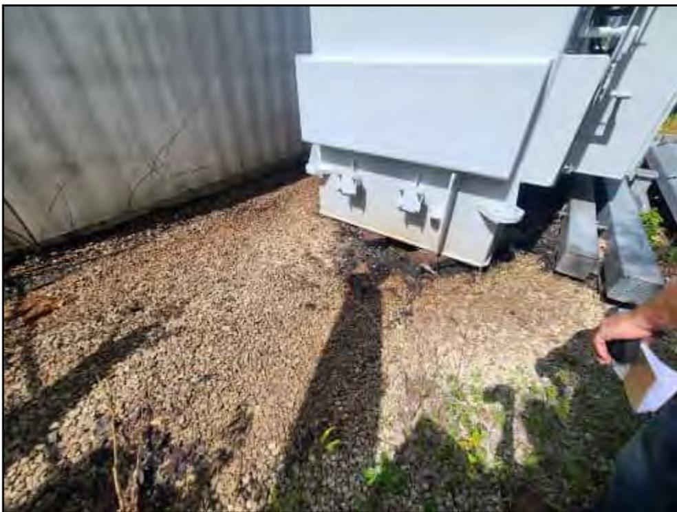
View of outdoor bone yard storage area (17) leaking transformer
