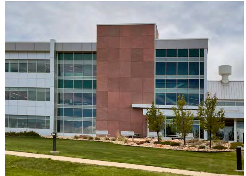
Building 3 Façade, Contemporary Building Materials
