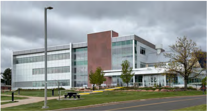
Building 3: Liquifier Building
