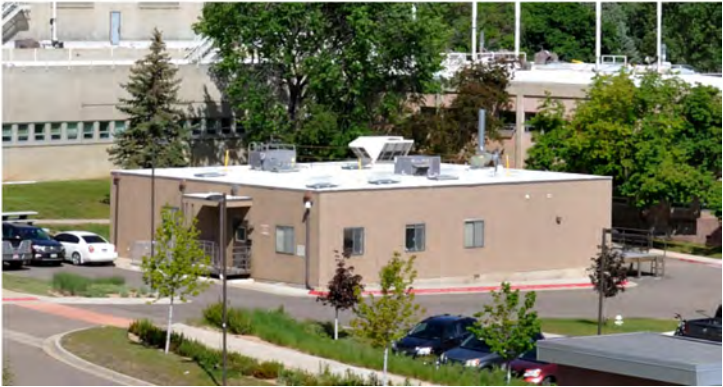
Building 2A: Cryogenic Annex
