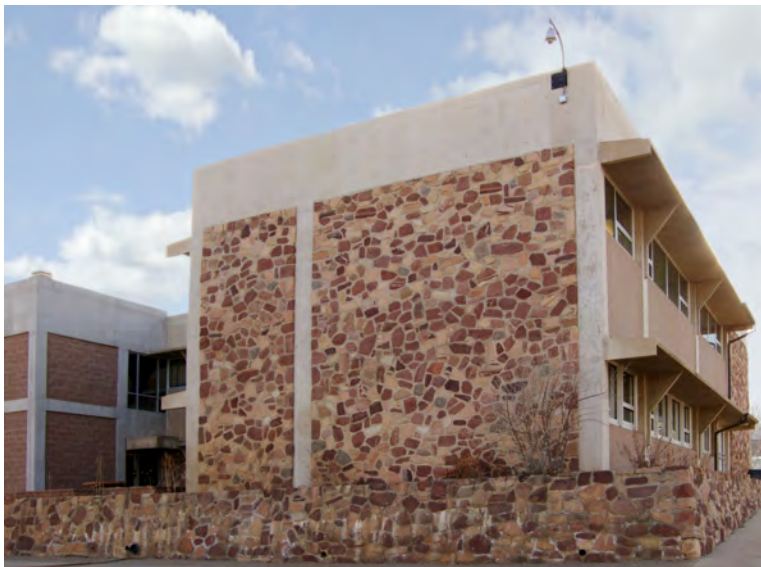
Typical Campus Lyons Sandstone Façade Materials
