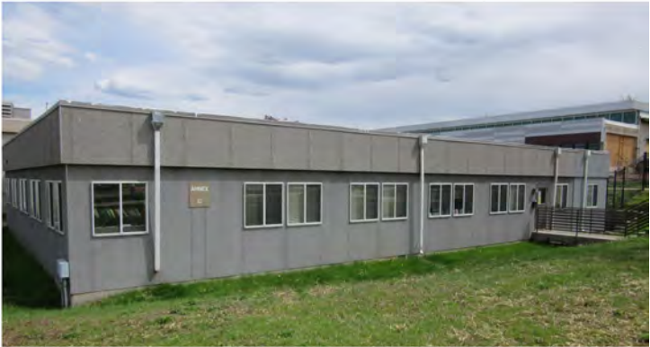
Building 1: Annex D
