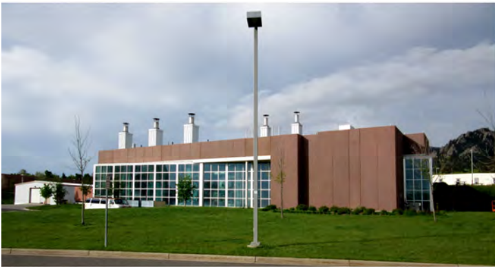
Building 42: Central Utility Plant
