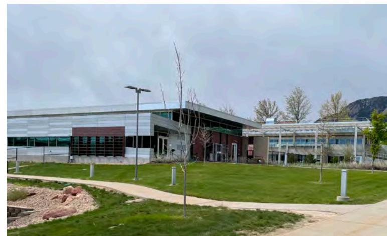
Building 1, Wing 3 and Wing 5
