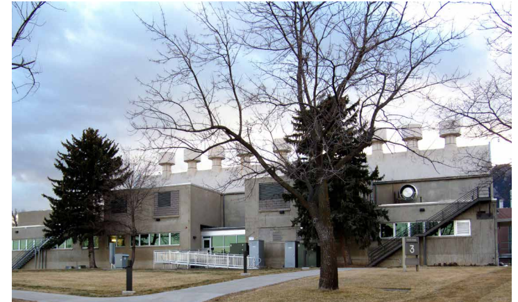
Building 3: Liquifier Building
