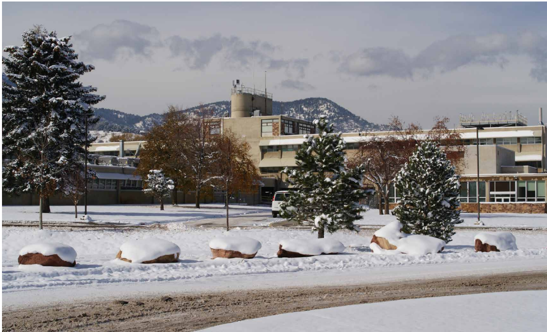
Building 1: Radio Building
