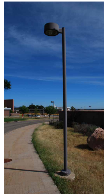
Existing solar utility lights
