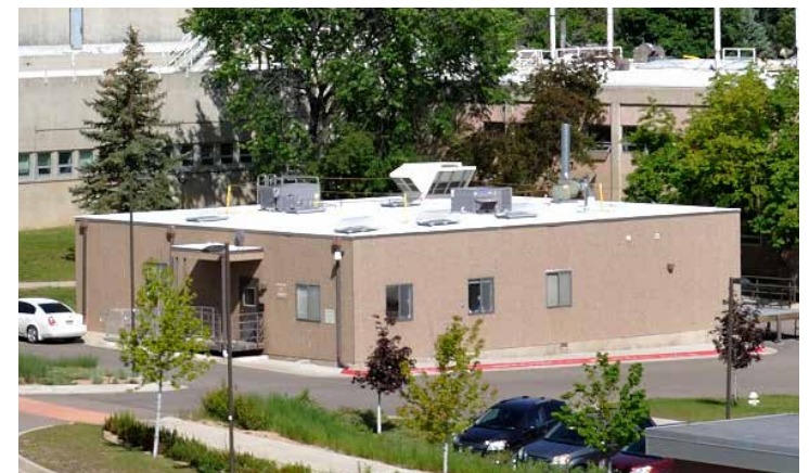
Building 2A: Cryogenic Annex
