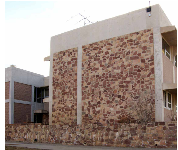
Exhibit 101: Typical Campus Lyons Sandstone Façade Materials
