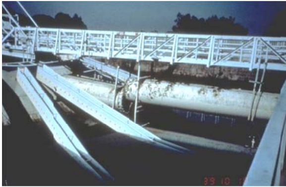
Figure 9-3. Santa Clara Valley Water District, Rinconada Water Treatment Plant Clarifier Launder Damaged due to Sloshing, 1989 Loma Prieta Earthquake (Courtesy of Don Ballantyne)
