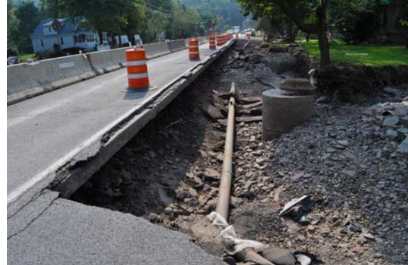
Figure 6-1: Road undercutting in the aftermath of Hurricane Irene (FEMA, Photo by Elissa Jun, 2011)
