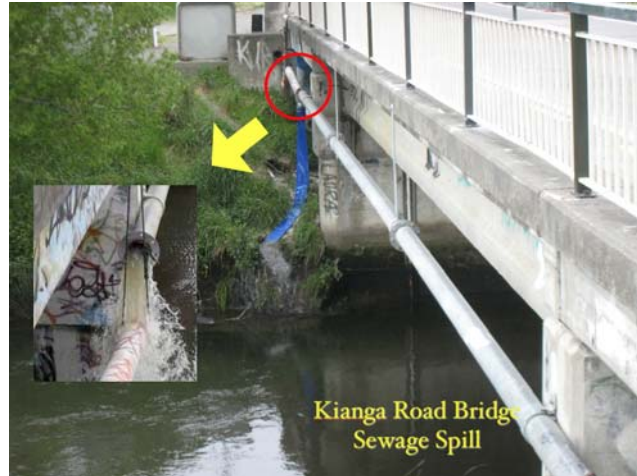
Figure 4-5: Example of Infrastructure Co-location (Source: Eidinger & Tang, 2014)
