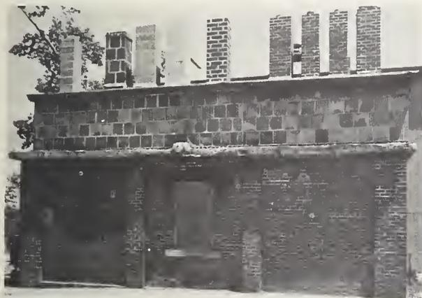
*A wide variety of masonry chimneys were studied in this building to evaluate their fire hazard potential and their draft-producing capabilities. The chimneys shown here differed in the size and shape of the chimney liner, the type of masonry unit, and the treatment of the air space between masonry and liner.*
