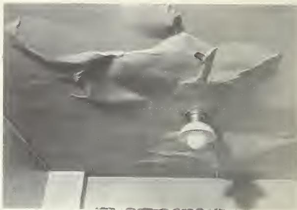
*Investigation of white-coat plaster has revealed how to avoid bulging and failure, such as shown here, caused by slow hydration and expansion of the magnesium in dolomitic limes.*
