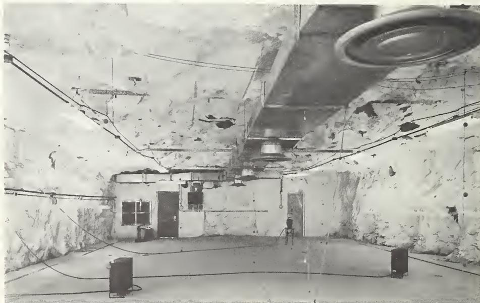
*A deep underground chamber, in solid rock, employed to conduct experimental studies of the initial and long-term heating, air-conditioning, and dehumidifying requirements of such chambers used to house personnel, communications equipment, and other heat-generating apparatus.*
