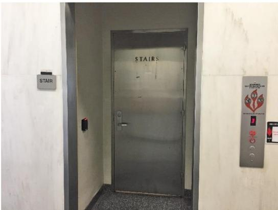
A stainless-steel door leads into the stairwell. Raised lettering spells out STAIRS in all capitals. Original hardware includes aluminum door knobs and stainless-steel modernist hinges. A lock set and lever handle have replaced original knobs at stair door.
