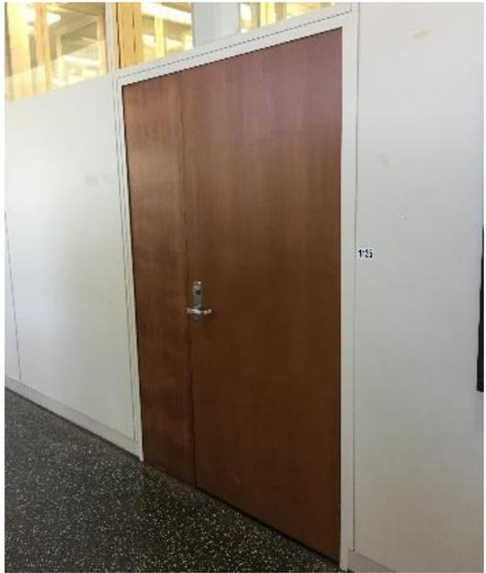
Office doors are single-leaf clad in walnut veneer. A wood panel with matching veneer is inserted to the left of the door. Original hardware includes aluminum door knobs and stainless-steel modernist hinges. A lock set and lever handle have replaced original knobs at most doors.
