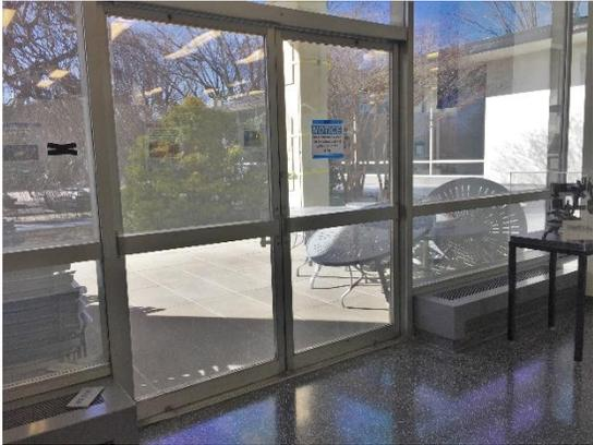
Aluminum and glass curtain wall systems extend from masonry columns at the east and west ends to the central stair core. Large rectangular lites are arranged vertically over smaller rectangular lites arranged horizontally. Double-leaf, full-lite doors are centered in both the east and west spans of curtain wall. A push bar visually divides the single lite at each door. The push bar is attached at either end to the stiles and does not bisect the lite.
