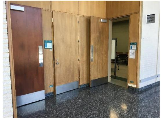
The typical door into the education block from the east and west corridors is a wood-veneer door with special stainless-steel hinges. The original doors had aluminum knobs but these have been replaced with aluminum door pulls and push plates. The wood door is missing from corridor access to the southwest office block.
