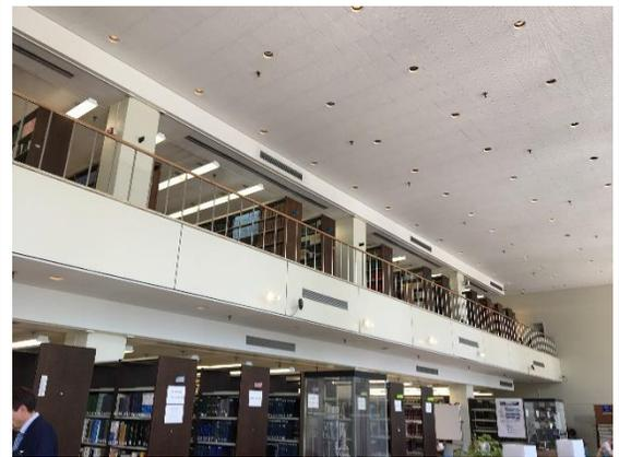
The mezzanine level runs the full length of the Library east to west and approximately two-thirds the width north to south. The face of the mezzanine is finished with plaster panels. An extruded aluminum air diffuser is centered in every third plaster panel. The stainless-steel balusters and American walnut handrail match those of the monumental spiral stair.
