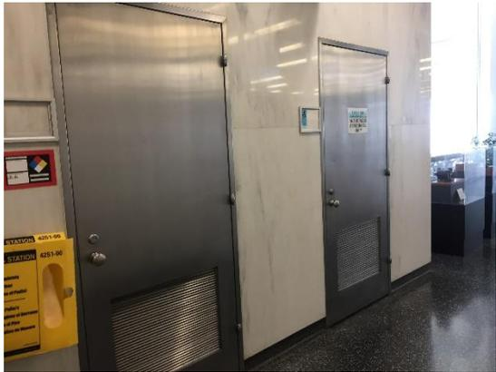
Utility closet doors are stainless steel with a louvered vent. Original hardware includes aluminum door knobs and stainless-steel modernist hinges.
