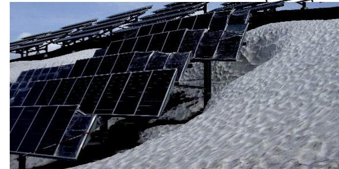
MW system +2000 m a.s.l. buried under several meters of snow in early Spring 2019.
