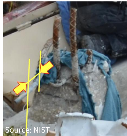
3 Position of Reinforcement Cage within Columns
