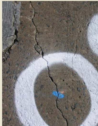
Vertical Cracking
