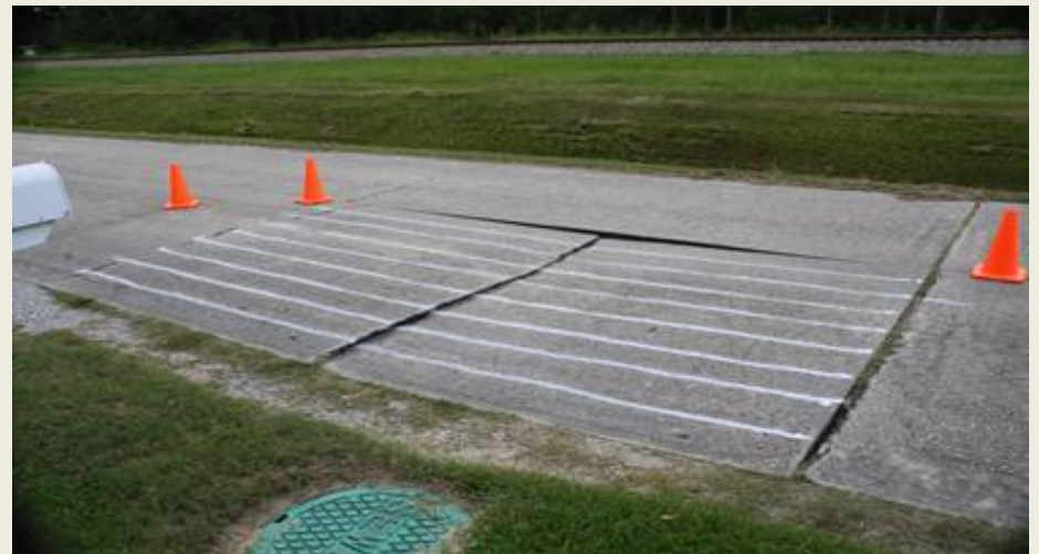
Leakage into adjacent brick-lined sewer created void under roadway, cracking of the concrete plate
