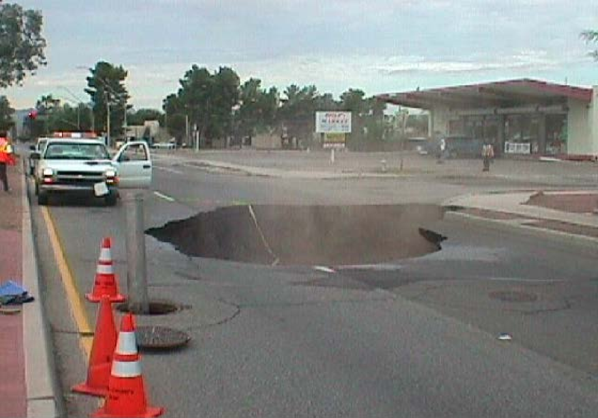
An Example of a Catastrophic Void
