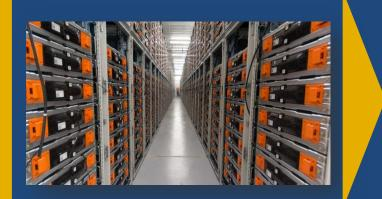
**Description:** Build one of the world's largest battery energy storage systems (BESS) (8MW for 4hr/32MWh), near Tehachapi wind farms to demonstrate 13 operational uses for energy storage including intermittent resource integration, operation and transmission benefits.
