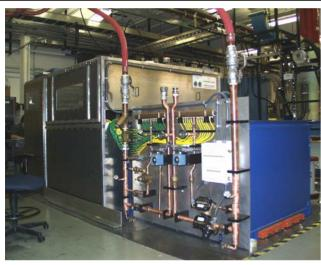
20 KHz, 10 MW Polyphase Pulsed Converter
