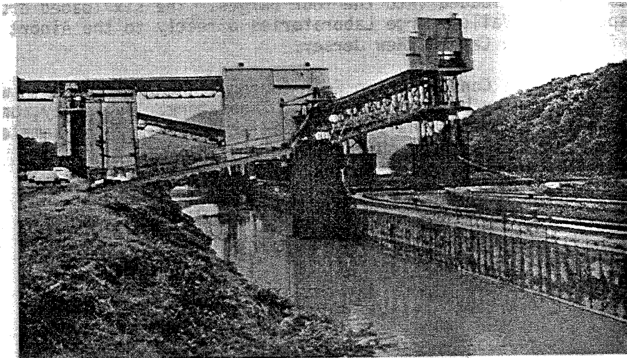
Figure B-3. Barge Loading System at Humphrey Plant.
