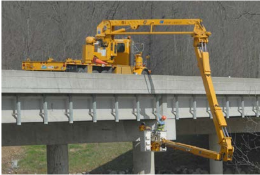
Visual Inspection (VI) Methods
