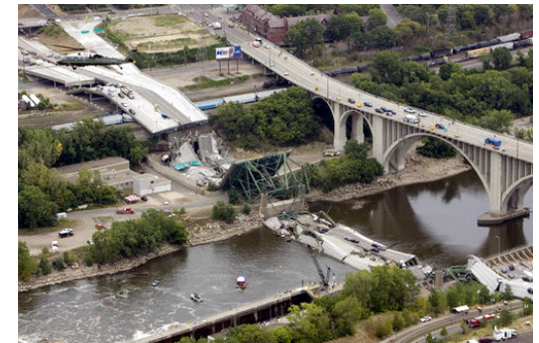
I35 Bridge, MN (13 deaths) August 1, 2007 [Under-designed gusset plates]
