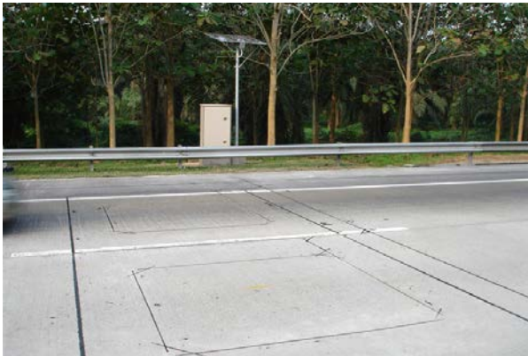
High-speed Weight in Motion [Michigan has 20+ WIMS Stations]
