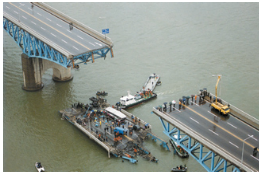
Songsu Bridge, Korea (31 deaths) October 21, 1994 [Poor design, construction and upkeep]
