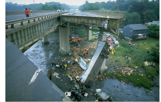
Mianus Bridge, CT (3 deaths) June 28, 1983 [Corrosion induced plate movement]
