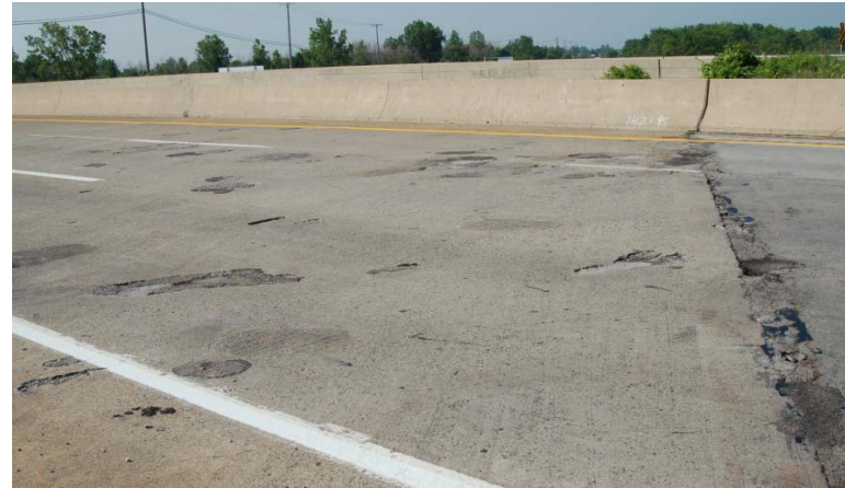
North Span Severely Cracked
