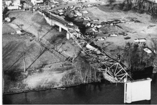
Silver Bridge, OH (46 deaths) December 15, 1967 [Stress corrosion cracking in eyebar]
