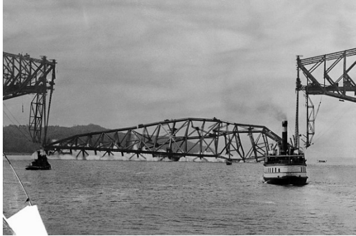
Quebec Bridge, Canada (95 deaths) September 11, 1916 [Inadequate capacity]
