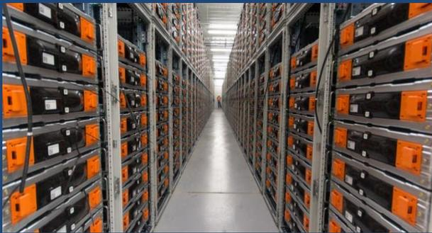
**Description:** Build one of the world's largest battery energy storage systems (BESS) (8MW for 4hr/32MWh), near Tehachapi wind farms to demonstrate 13 operational uses for energy storage including intermittent resource integration, operation and transmission benefits.
