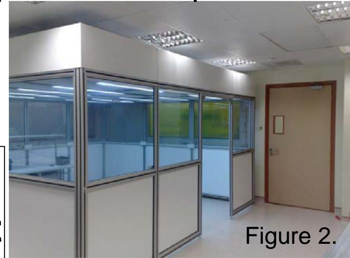
Figure 2. Exterior Hard wall clean lab space for new mass spectrometer
