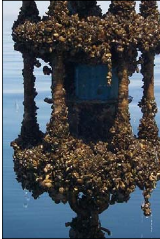
Zebra mussels clog a water intake pipe
