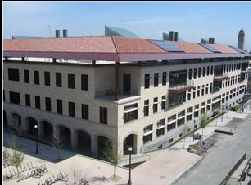
Supply Chain Fragmentation: Y2E2 Bldg.
