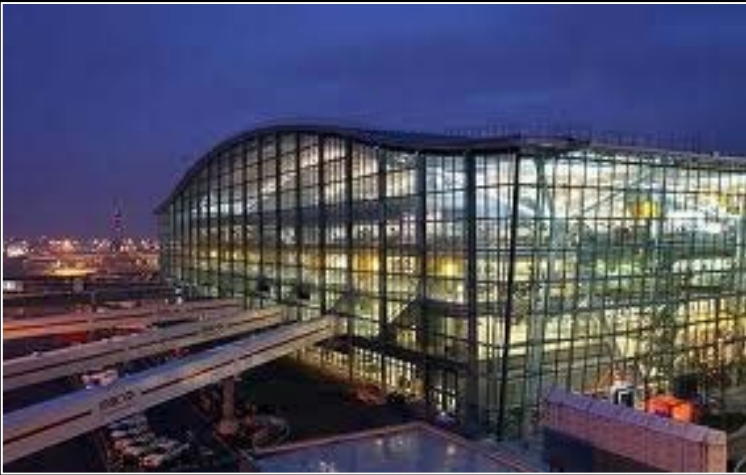
Heathrow Terminal Five
