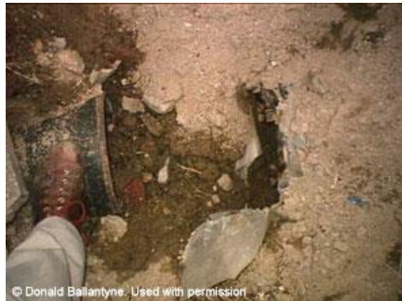
Figure 16-10: Ground cracking (left) and joint separation in ductile iron pipe (right) due to liquefaction during 1995 Kobe Earthquake
