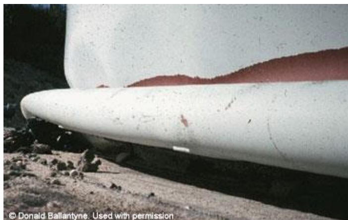
Figure 16-8: Steel tank elephant's foot buckling in 1994 Northridge Earthquake
