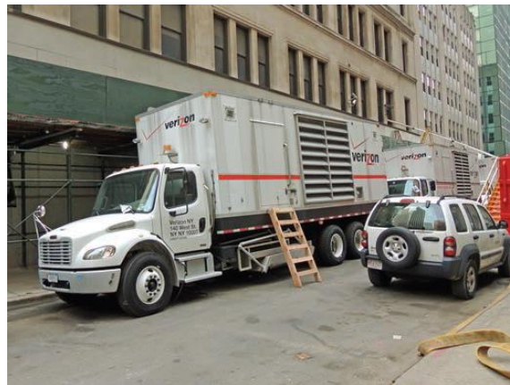
Figure 15-3: Large standby portable power unit used when basement generators failed [Source: FEMA 2013]
