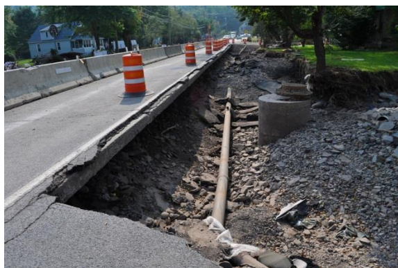
Figure 13-1: Road undercutting in the aftermath of Hurricane Irene (Source: Photo by Elissa Jun [FEMA 2014a])
