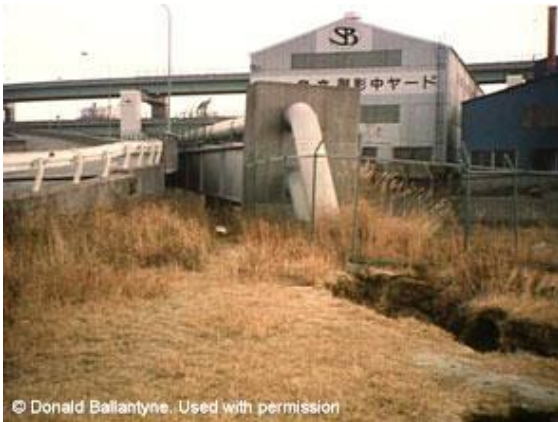
Figure 16-10: Ground cracking (left) and joint separation in ductile iron pipe (right) due to liquefaction during 1995 Kobe Earthquake
