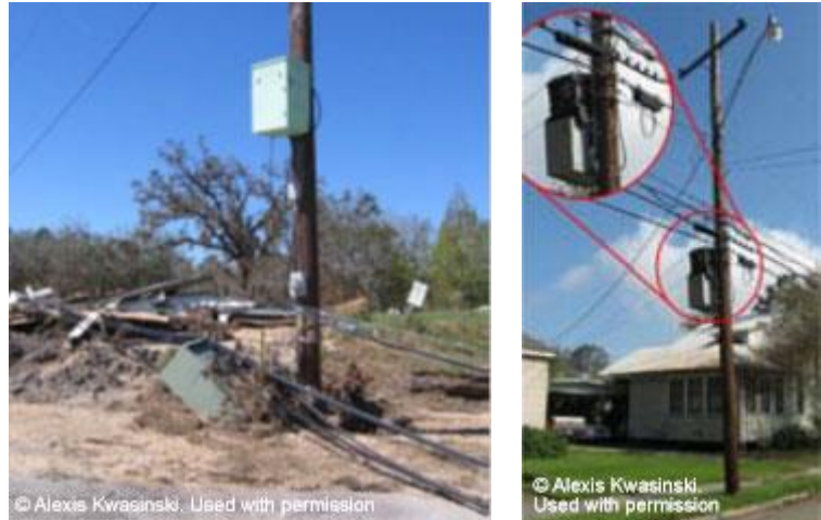
Figure 15-6: Placement of UPS systems is an important consideration for resilience and periodic maintenance.
