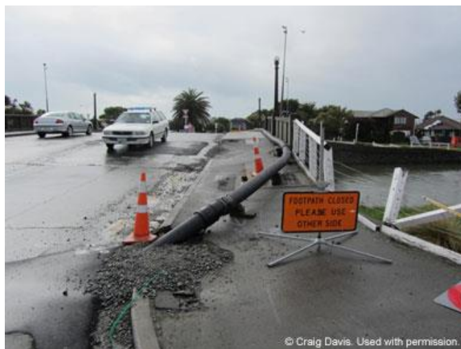
Figure 11-6: Example of infrastructure co-location
