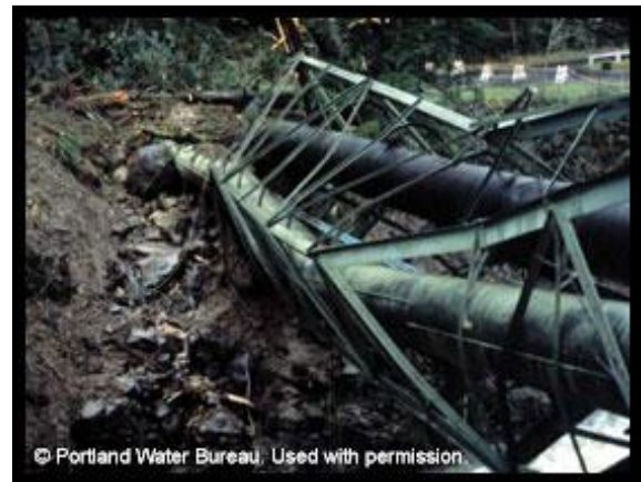
Figure 16-2: Water transmission pipeline bridge damaged by landslide
