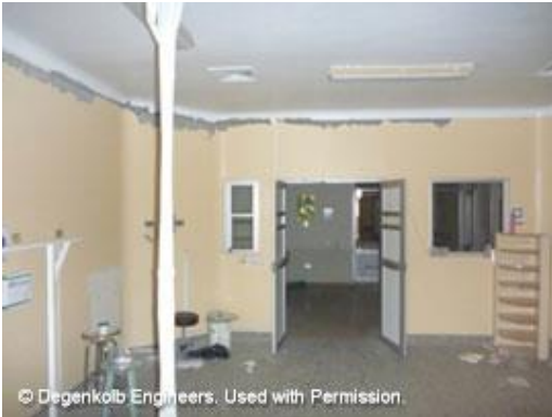
Figure 12-2: Non-structural damage to interior finishes following an earthquake event
