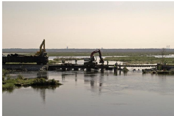
Figure 13-4: A railroad bridge in New Orleans was washed out by flooding during Hurricane Katrina. (Source: Photo by Marvin Nauman [FEMA 2014c])
