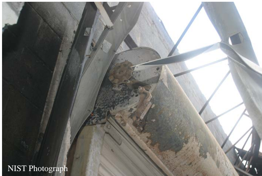
Figure O-9. East side of breezeway roll-up fire door mechanism.
