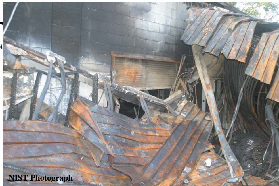
Figure O-55. Main showroom roll-up fire door looking toward rear of east showroom. Door identified as roll-up fire door #7 in Figure O-1. Door only closed about one-third of the way down during the fire.
