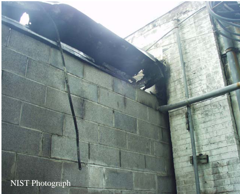
Figure I-4. Area on the rear wall of main showroom that was filled in with concrete blocks.
