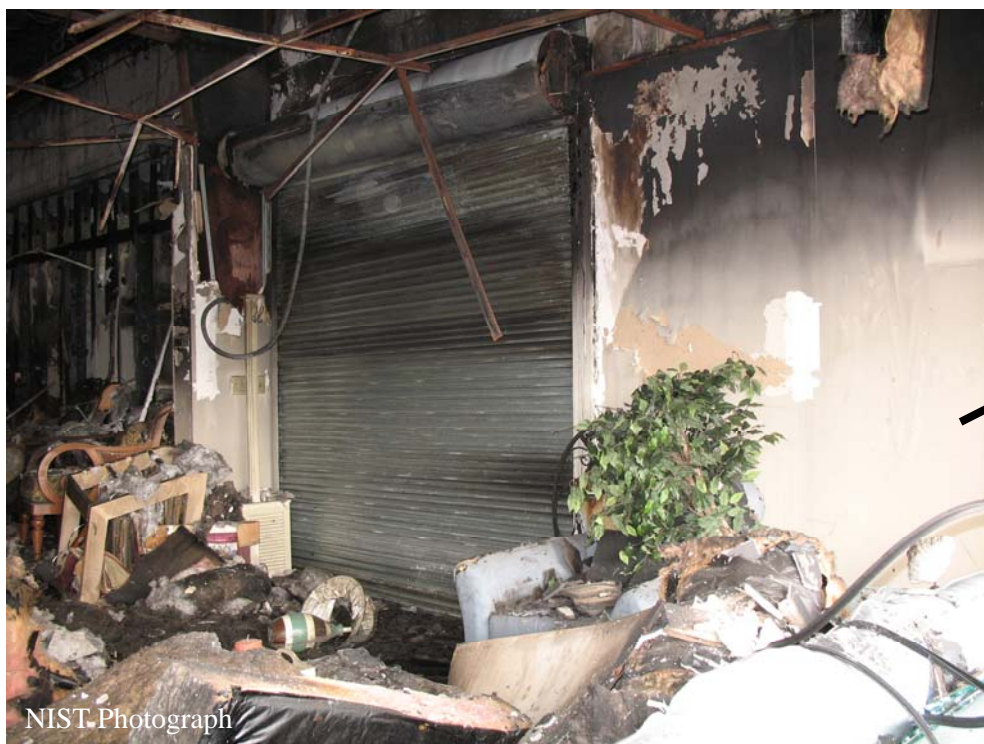
Figure O-33. Main showroom roll-up fire door looking toward front of main showroom. Door identified as roll-up fire door #5 in Figure O-1.
