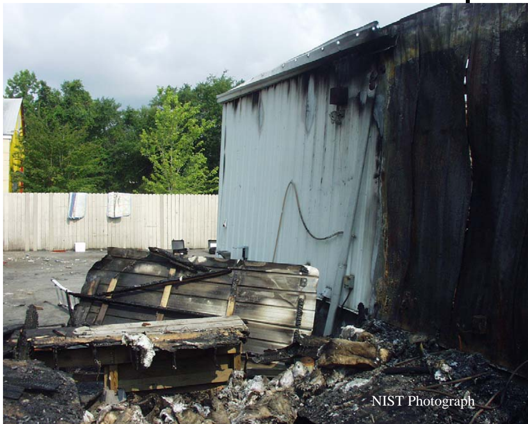
Figure C-16. Loading dock floor in foreground. Rear wall of west showroom on right of photograph. Darker section of rear wall was inside the enclosed loading dock area. Lighter portion of wall was outside enclosed loading dock.
