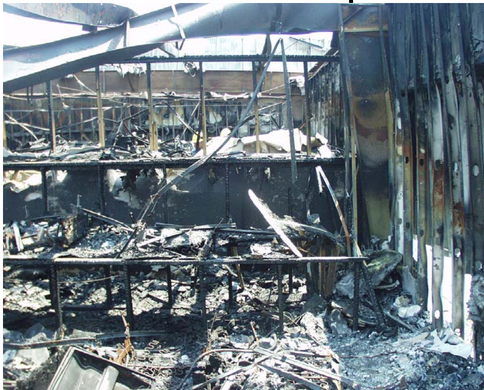
Figure E-18. Interior view along west wall of west showroom. Wood supports for two level display platforms visible in center of photo. Vertical wood studs of partition wall visible behind display platform remnants. Steel I-beam column and roof support also visible on right and top of photo.
