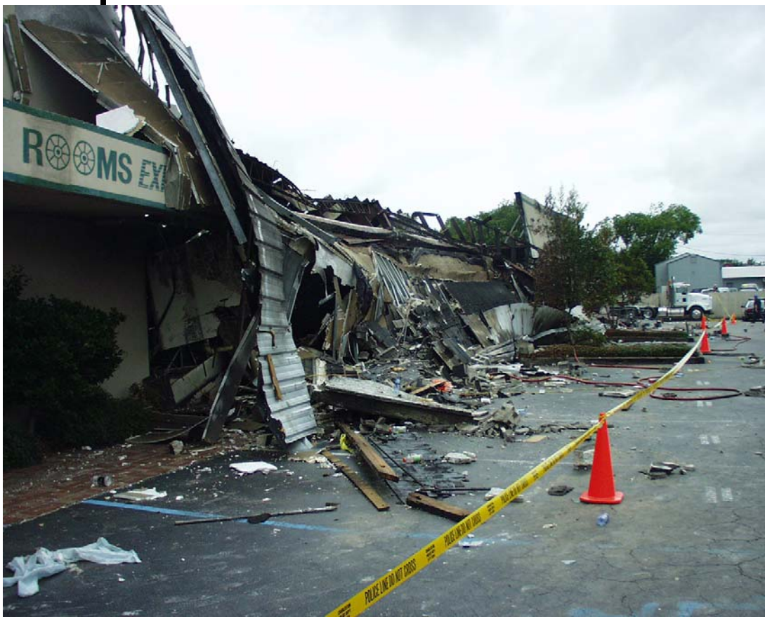
Figure D-3. Front of main showroom. Facade and parapet wall collapsed into parking spaces.
