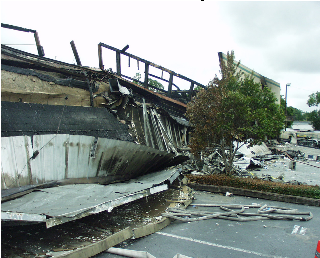
Figure D-2. Front of main showroom. Façade and parapet wall collapsed into parking spaces.
