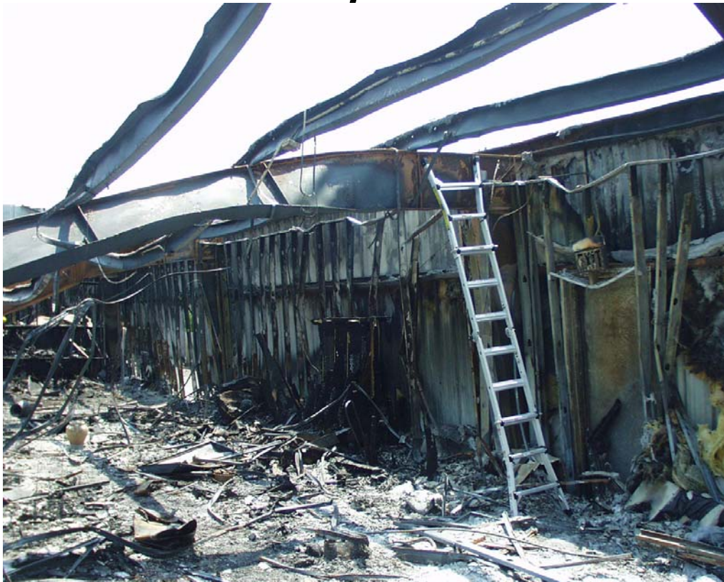
Figure E-17. Interior view of north-west corner of west showroom. Sagging I-beam and roof Z-channel visible in photo. Exit door in west wall near front of showroom visible to right of ladder.
