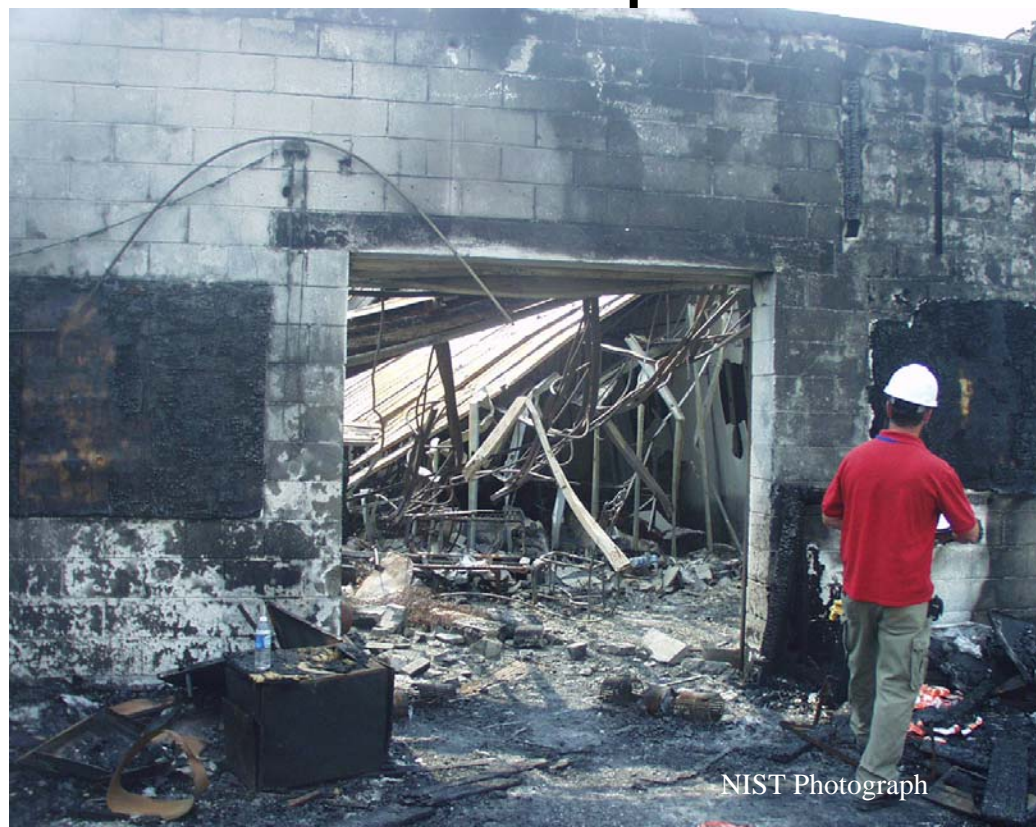
Figure C-9. Non-fire roll-up door between loading dock and holding area as viewed from loading dock.
