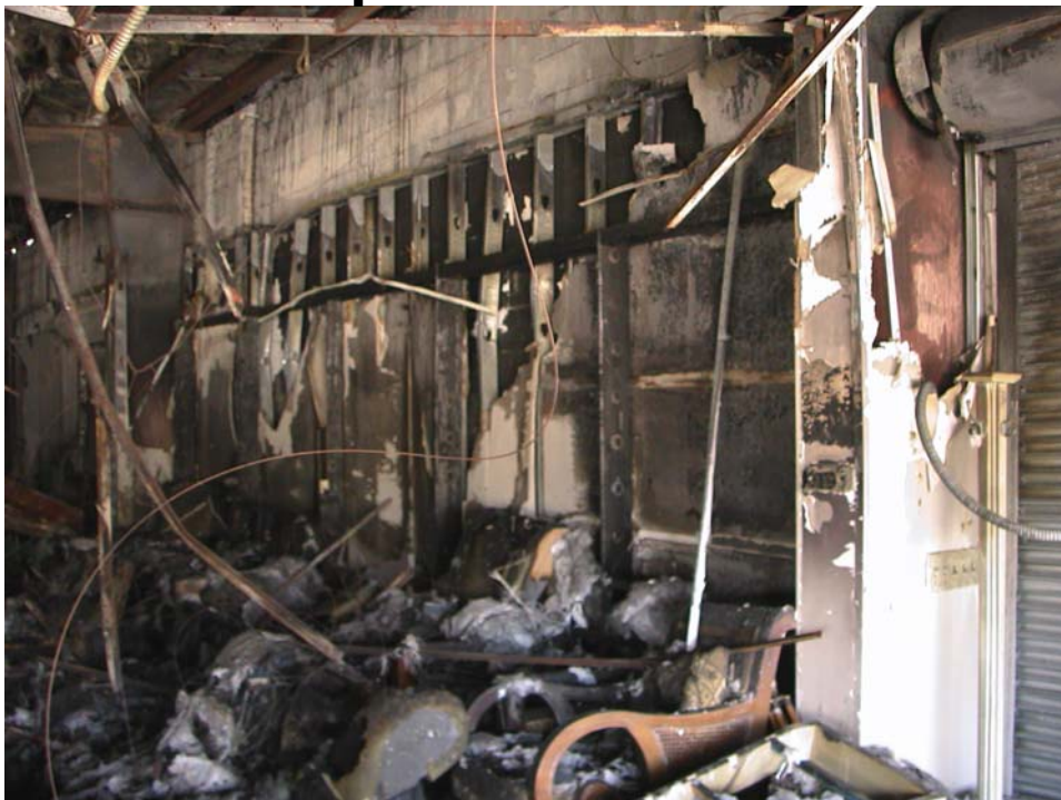
Figure F-19. Interior of east showroom. Closed roll-up fire door visible on right of image.
