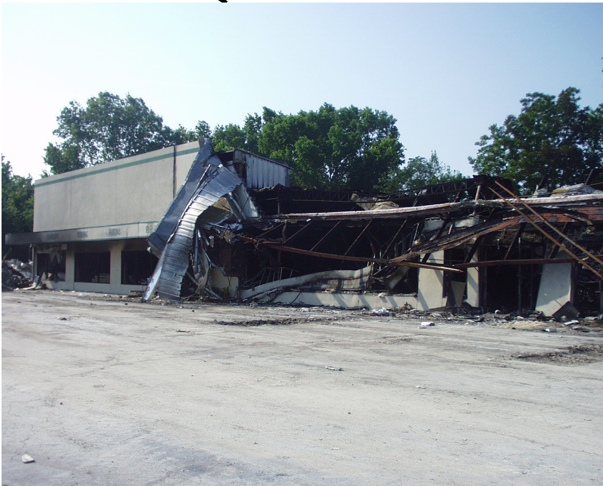
Figure D-13. Front of main showroom after removal of collapsed façade. Façade and parapet wall of east showroom still in place.
