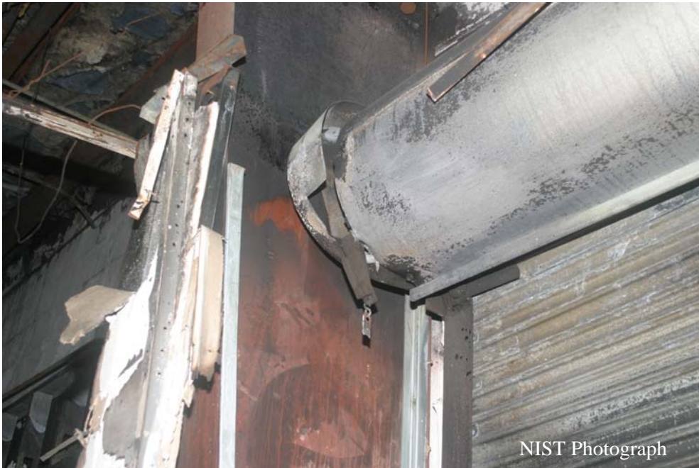
Figure O-37. South side of operating mechanism for roll-up fire door #5. Portion of fusible link visible in center of photo.
