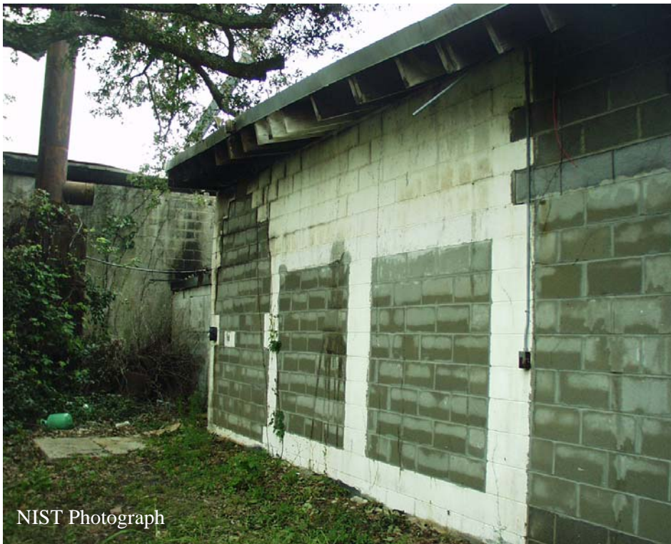
Figure I-8. Openings on the rear wall of main showroom that were filled in with concrete blocks.
