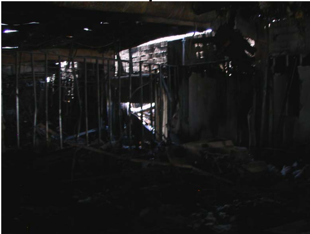
Figure F-16. Interior view of east showroom looking toward partially closed roll-up fire door. Metal studs of rear partition wall visible in left-center background of photo.
