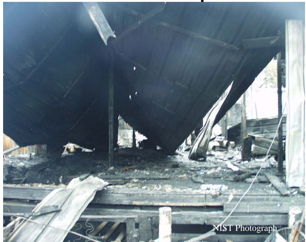
Figure C-3. Remains of center portion of west wall of loading dock. Line of studs on right supported 2.7 m (9 ft) high section while line of studs in left center of image supported 3.7 m(12 ft) high section.
