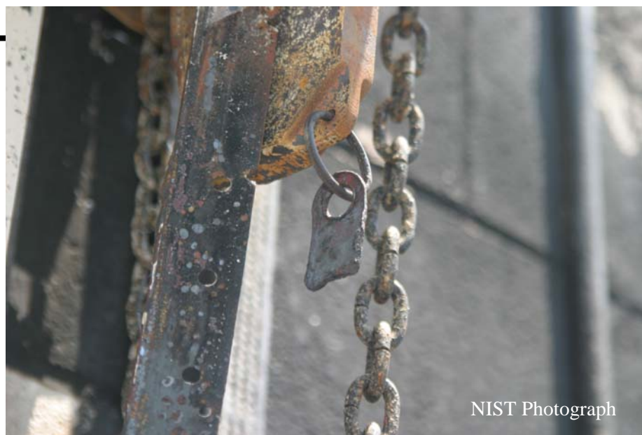
Figure O-24. South side of operating mechanism for roll-up fire door #3. Lower portion of fusible link visible.
