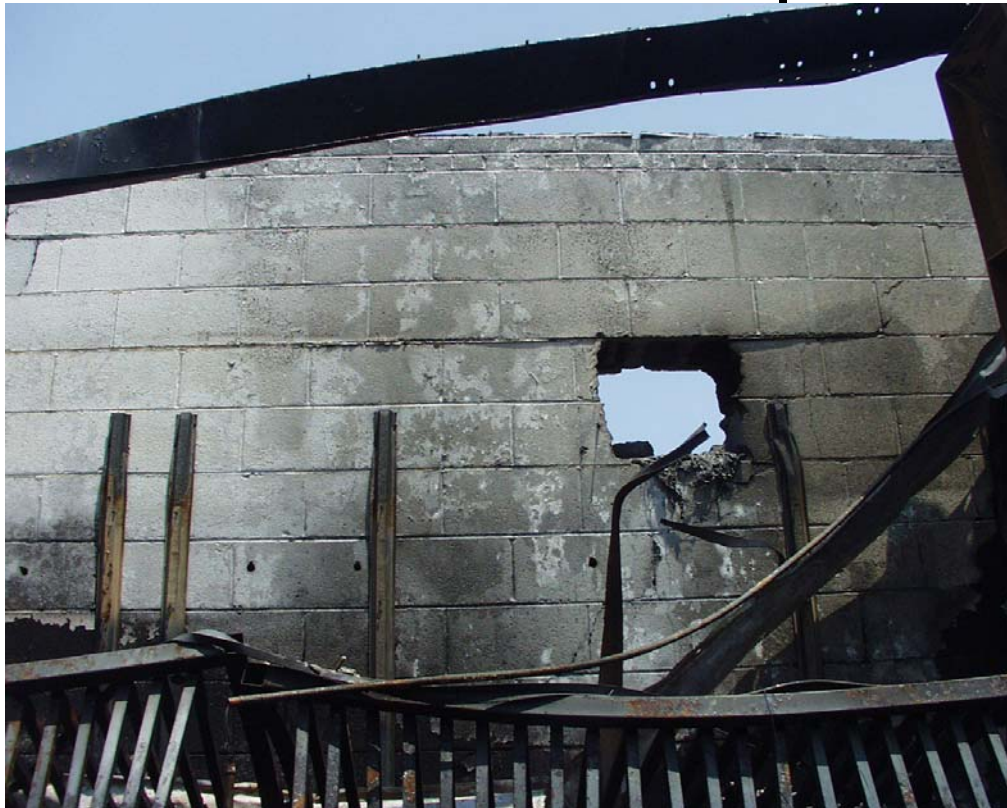
Figure E-26. Interior of west showroom above drop ceiling looking toward main showroom. Open hole, approximately 0.5 m ( 1.5 ft) x 0.5 m (1.5 ft) opening through concrete block wall. This hole may have allowed smoke to move from interstitial space above drop ceiling in main showroom to the interstitial space above the drop ceiling in the west showroom.
