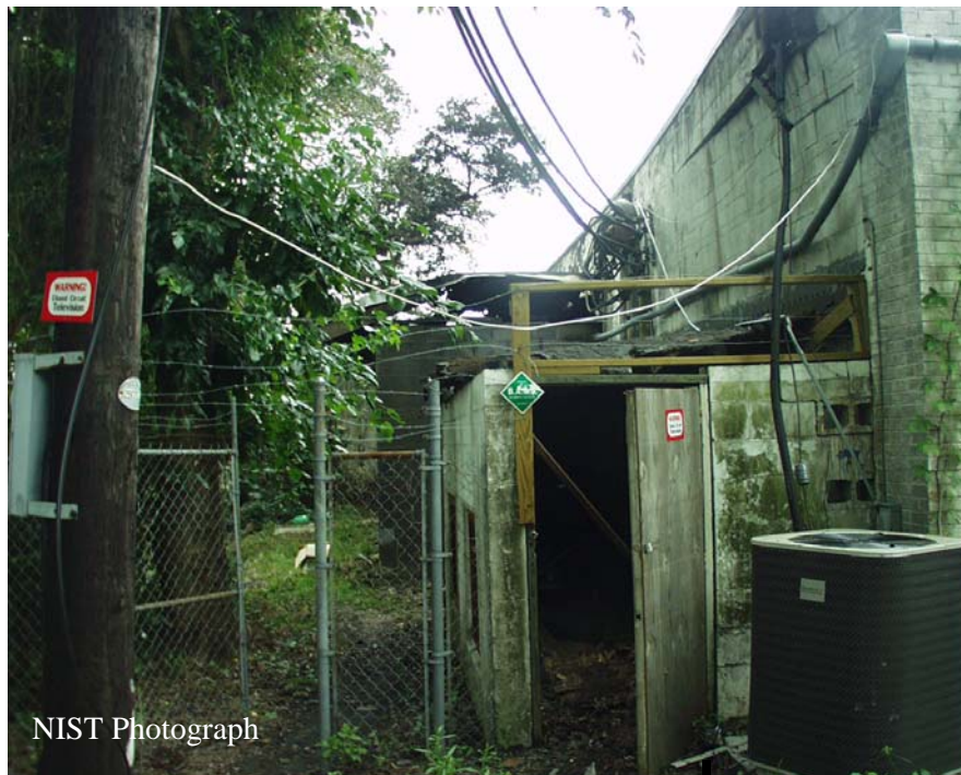
Figure I-3. Rear wall of main showroom. When structure was used as a grocery store, refrigeration equipment was probably located in enclosed area attached to rear wall of main showroom. There did not appear to be a door opening between enclosed area and main showroom.
