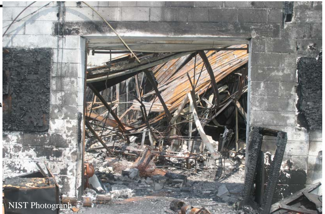
Figure O-12. Non-fire roll-up loading dock door looking toward rear of main showroom.
