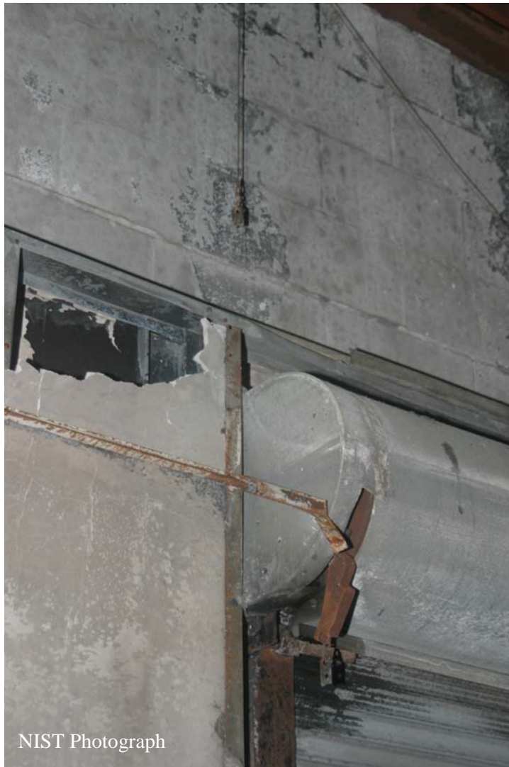
Figure O-46. South side of operating mechanism for roll-up fire door #6. Portion of fusible link visible in center of photo.
