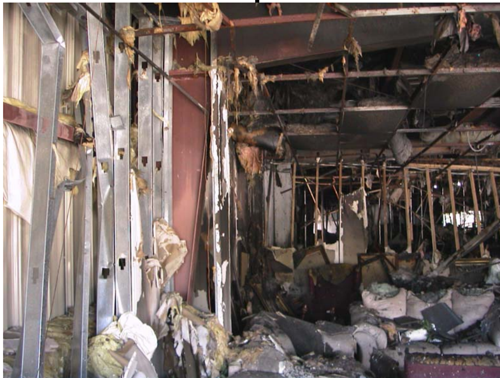
Figure F-21. Interior of east showroom looking along east wall toward rear of showroom. Exterior metal wall attached to exterior side of horizontal channel. Metal studs attached to inside face of horizontal channel. Gypsum wall board was installed over metal studs to form interior wall of showroom. Metal stud/gypsum wall appeared to extend approximately 0.3 m ( 1 ft) above drop ceiling along east wall. Reddish-brown steel I-beam column and roof joist also visible in photo.
