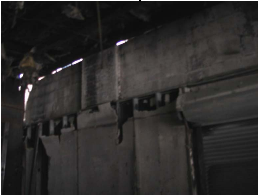
Figure F-20. Interior view of east showroom looking toward main showroom. Concrete block wall was originally exterior wall of grocery store. Gypsum wall board attached to metal stud which were attached to concrete block wall. Metal studs/gypsum wall board extended up to drop ceiling, but not above drop ceiling.
