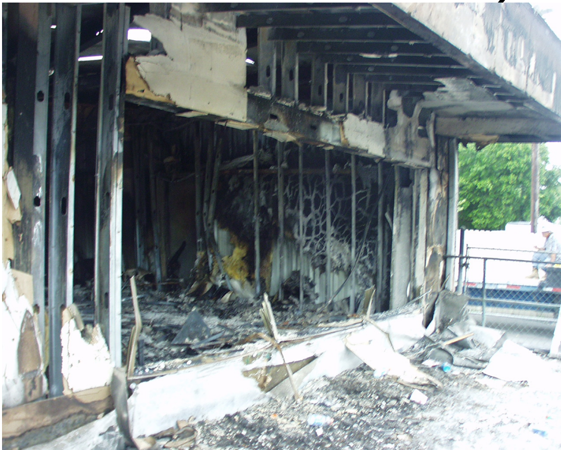
Figure E-3. Exterior view of front of west showroom. Metal stud walls visible.
