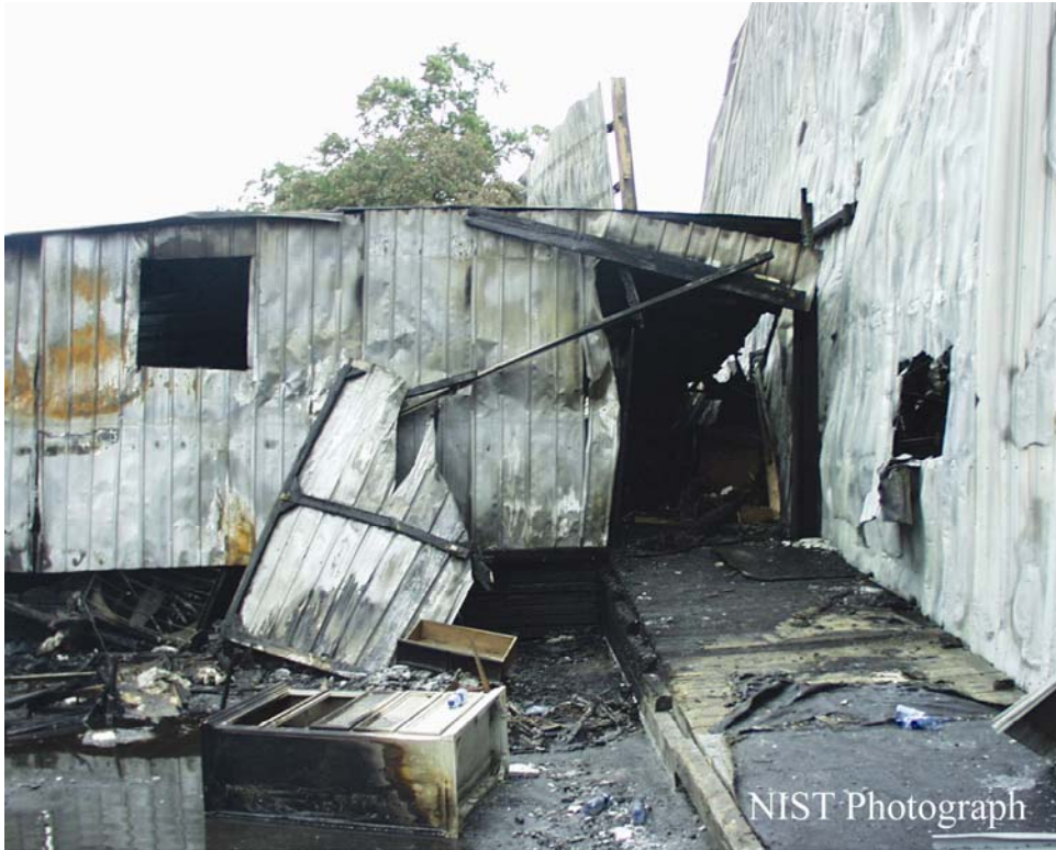
Figure K-9. Photograph showing the outside of the loading dock. This was identified as the area of fire origin.
