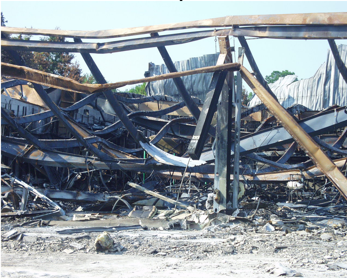
Figure E-12. Exterior view of west showroom looking into enter-front portion of showroom. Roof Z-channel and I-beam supports sagged to within 1m (3.3 ft) of showroom floor.
