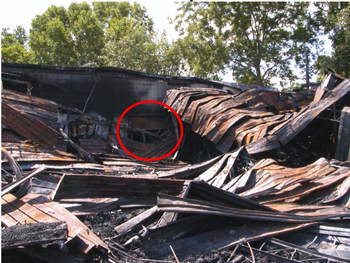
Figure D-24. Interior of main showroom looking toward east wall. Partially closed roll-up fire door circled.
