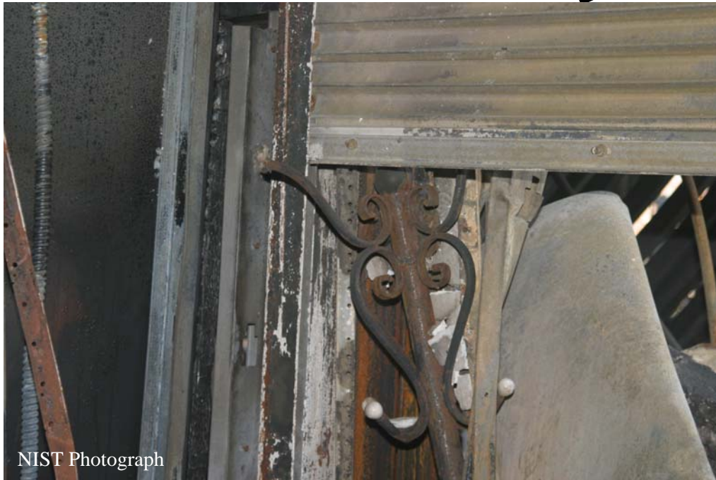
Figure O-54. Main showroom roll-up fire door looking toward rear of main showroom. Movement of door impeded by coat rack. Door only closed about one-third of the way.
