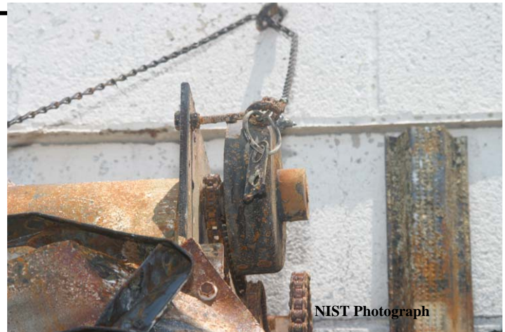
Figure O-25. South side of operating mechanism for roll-up fire door #3. Upper portion of fusible link visible in center of photo.
