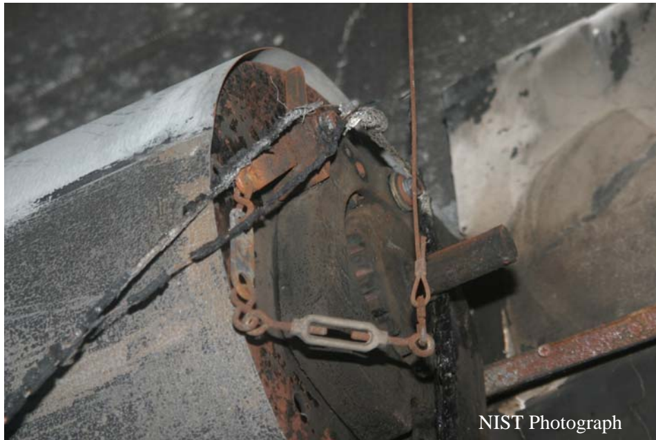
Figure O-36. North side of operating mechanism for roll-up fire door #5.
