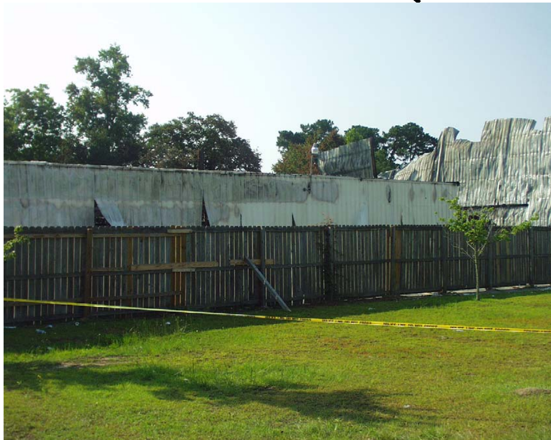
Figure E-6. West wall of west showroom. Discoloration patterns due to exposure to high temperatures visible on metal siding. Front section of west showroom displayed more discoloration than rear section of west showroom. Wooden fence separates furniture store from adjacent property.
