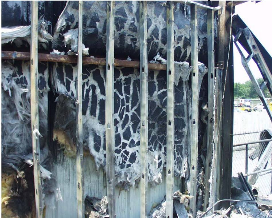
Figure E-31. Interior of west showroom looking at west wall near front of store. Exterior metal wall attached to exterior side of horizontal channel. Metal studs attached to inside face of horizontal channel. Gypsum wall board was installed over metal studs to form interior wall. Metal stud/gypsum wall appeared to extend approximately 0.3 m (1 ft) above drop ceiling along west wall. Fiberglass insulation is visible between metal studs and exterior metal siding.
