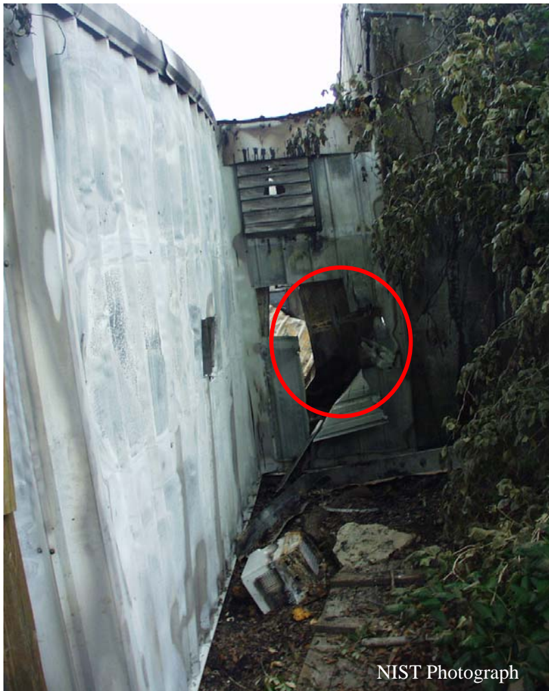
Figure H-3. Intersection of walls of two repair shops with rear wall of main showroom. Trapped employee was extracted from opening in metal siding visible in center of photo (circled area). Air conditioner which had been mounted in rectangular opening in wall fell out and was on ground below opening.
