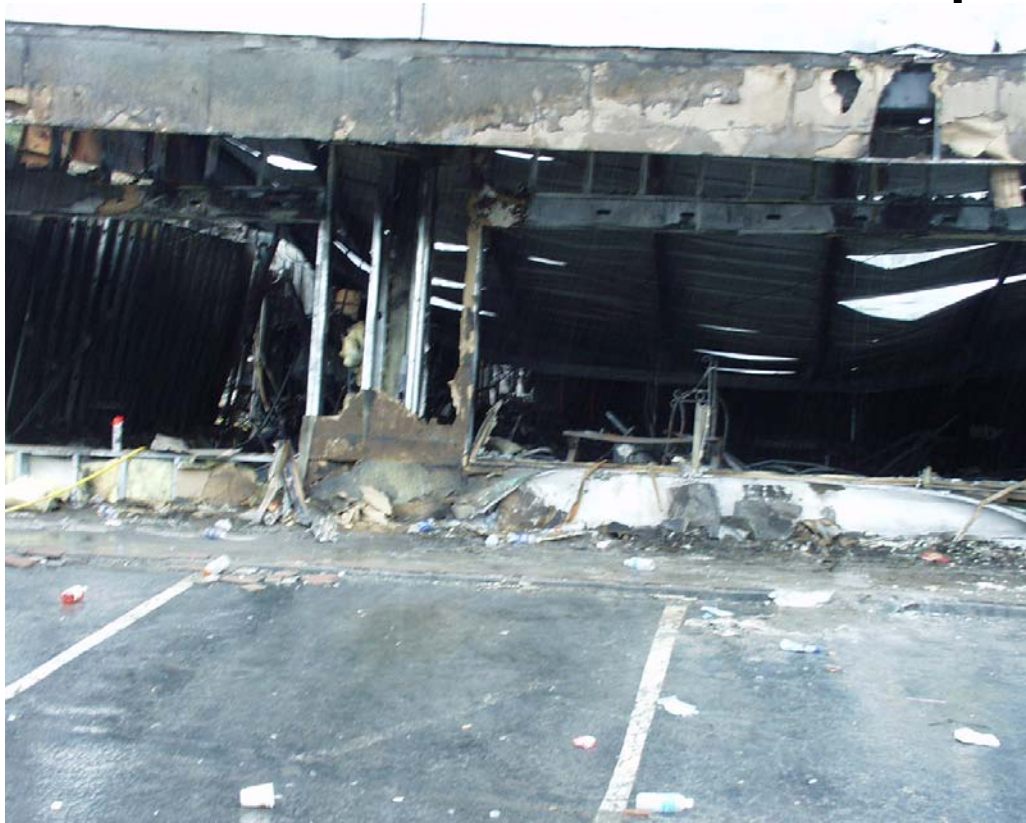
Figure E-2. Exterior of west showroom. Remains of east- and center-front window sections visible.
