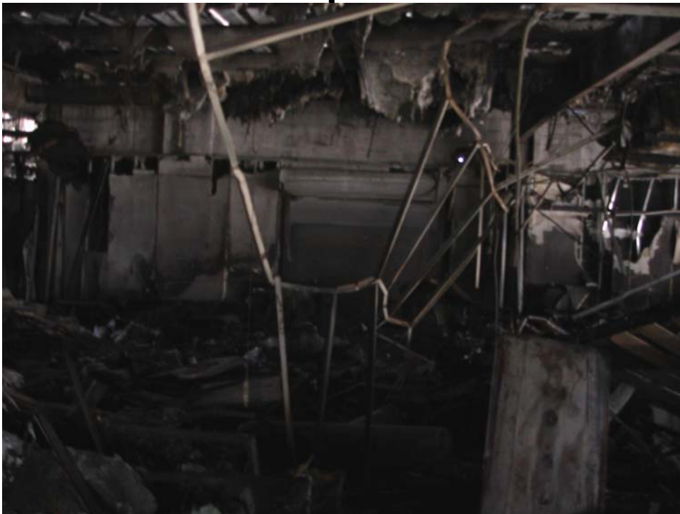
Figure F-15. Interior of east showroom looking toward main showroom. Closed roll-up fire door visible in center of photo. Photo displays more damage from fire in this center section of east showroom.
