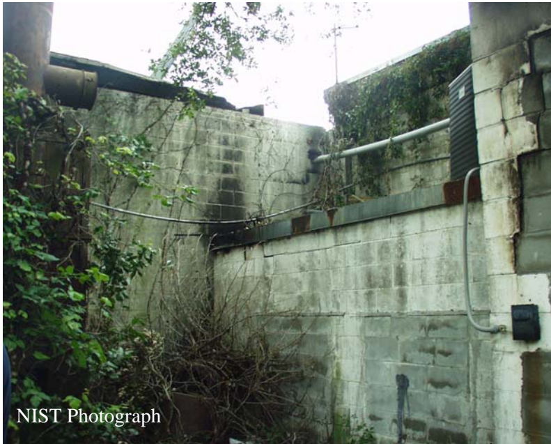
Figure I-11. Openings on the rear wall of main showroom that were filled in with concrete blocks. Incinerator visible in left of photograph.
