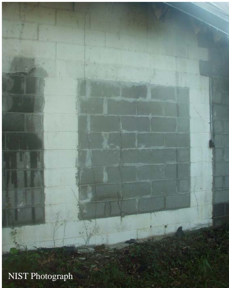
Figure I-9. Openings on the rear wall of main showroom that were filled in with concrete blocks.
