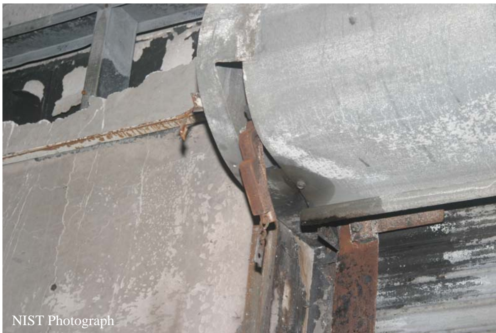
Figure O-45. South side of operating mechanism for roll-up fire door #6. Portion of fusible link visible in center of photo.
