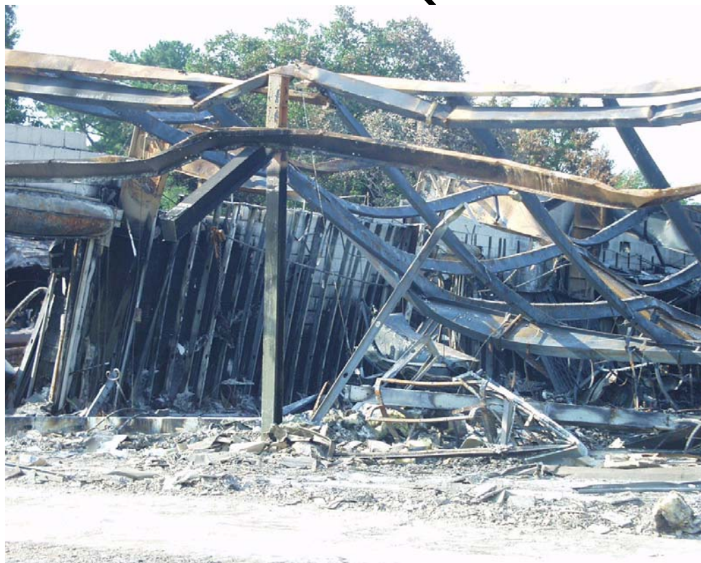
Figure E-13. Exterior view of west showroom looking into east-front portion of showroom. Metal stud wall attached to west wall of main showroom visible in center of photo. Open roll-up fire door partially visible at left center of photo.
