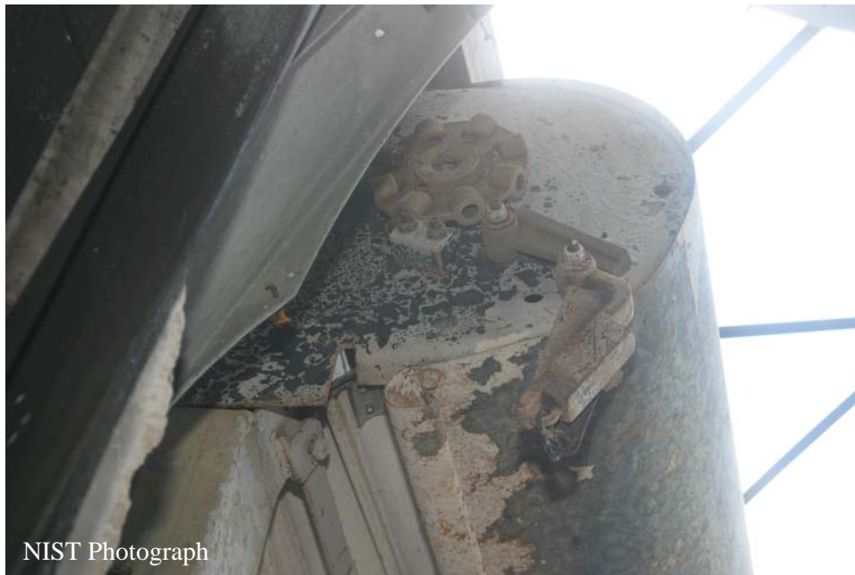
Figure O-10. East side of breezeway roll-up fire door mechanism.
