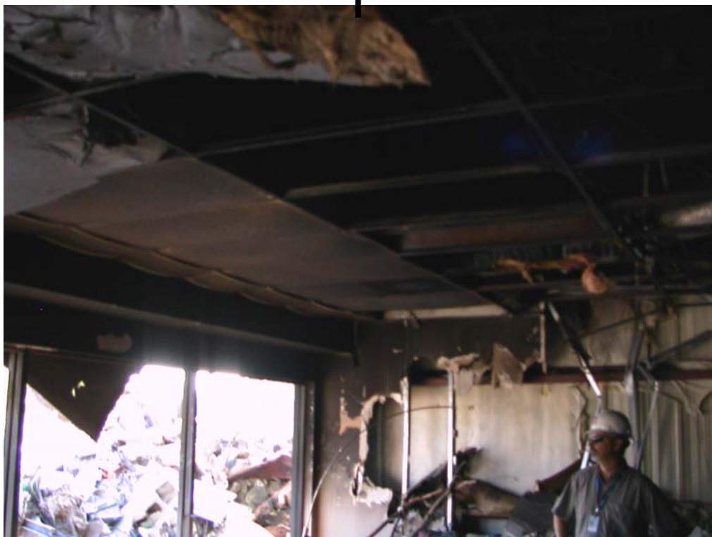
Figure F-17. Interior view of east showroom looking at drop ceiling. Exterior metal siding visible in center right of photo. Portions of gypsum wall board visible in center background of photo.
