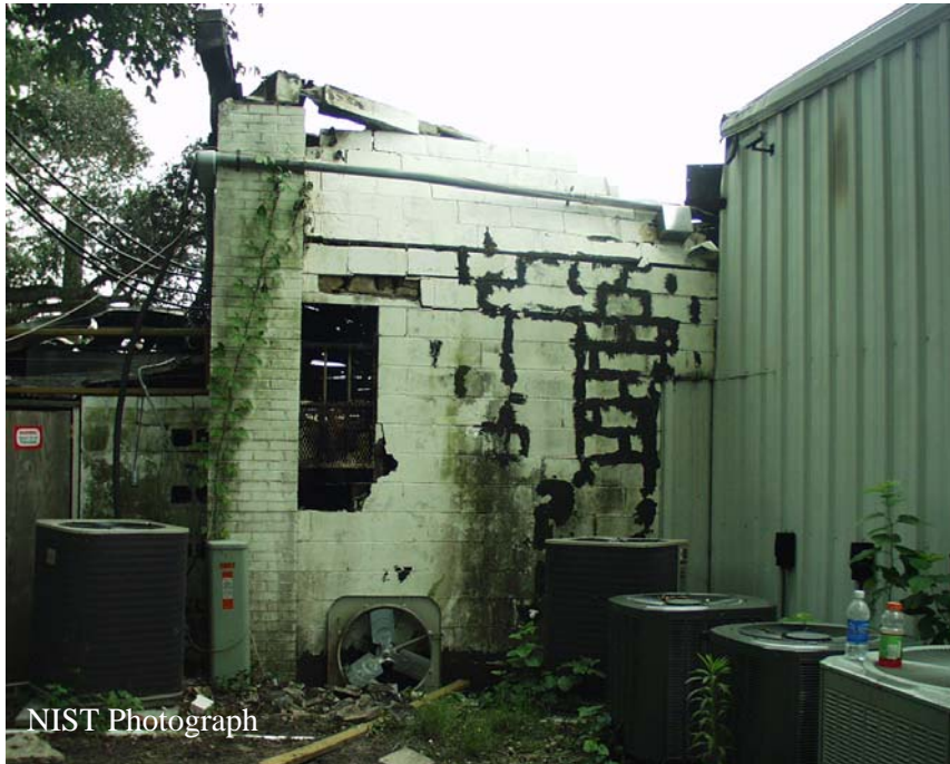
Figure I-2. Rear wall of store. Intersection of metal siding at rear of east showroom and concrete block wall at rear of main showroom.
