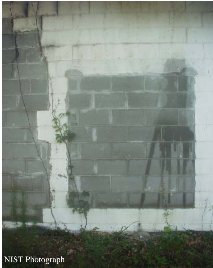
Figure I-10. Opening on the rear wall of main showroom that was filled in with concrete blocks.
