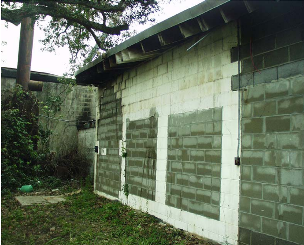
Figure D-7. Rear of main showroom. Openings in original wall have been filled in with concrete masonry blocks.
