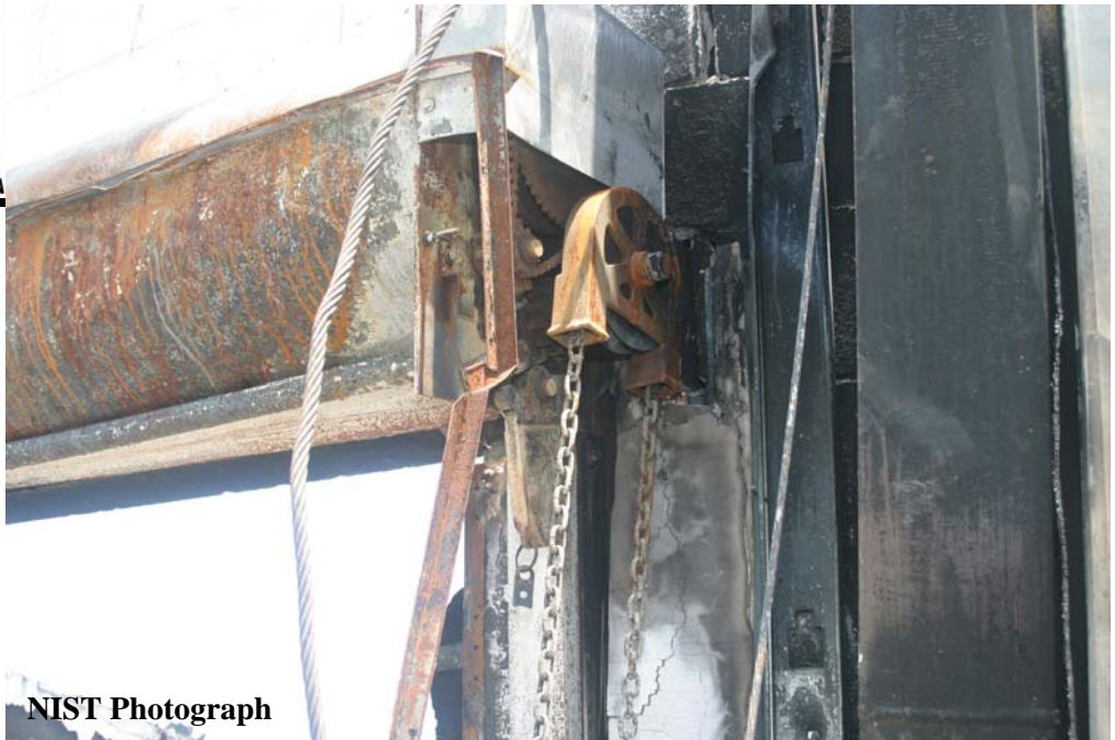
Figure O-17. South side of operating mechanism for roll-up fire door #4.
