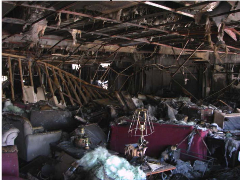
Figure F-14. Interior of east showroom looking toward main showroom. Closed roll-up fire door visible in center-right background. Partially closed roll-up fire door visible in center background. Photo displays less fire damage to furniture in front section of east showroom.
