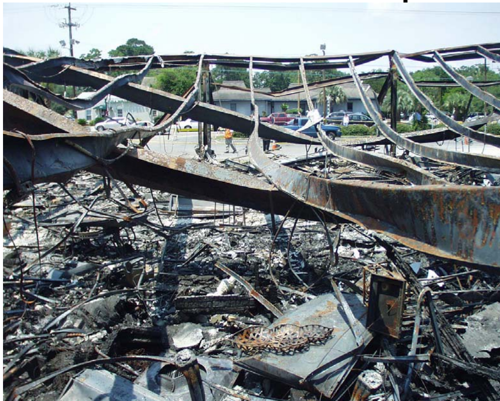
Figure E-30. Interior of west showroom looking toward front of showroom. Portions of two (left to right) I-beam steel supports and nine Z-channel roof supports are visible. Exposure to high temperatures caused I-beam and Z-channel to sag within 1m (3.3 ft) of showroom floor.
