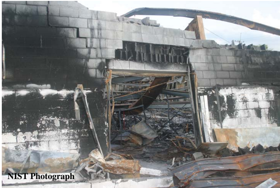
Figure O-28. Main showroom roll-up fire door looking toward middle of west showroom. Door identified as roll-up fire door #3 in Figure O-1.
