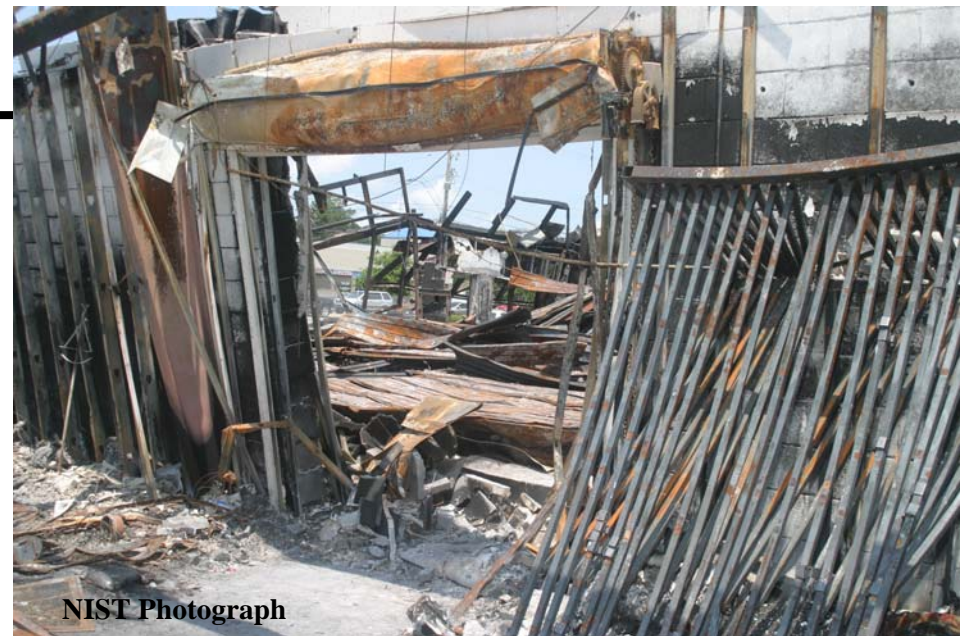
Figure O-22. Main showroom roll-up fire door looking toward middle of main showroom. Door identified as roll-up fire door #3 in Figure O-1.
