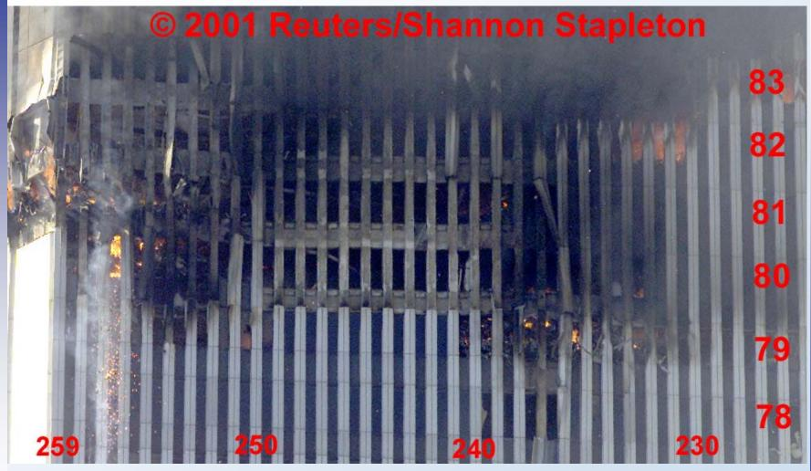
North Face of the South Tower. Image shows what appear to be portions of several floor slabs hanging across window openings on Floors 80, 81, and 82
