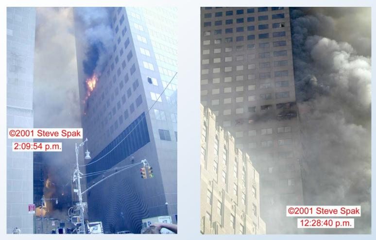
Fires in WTC 7—which began soon after WTC 1 collapsed—were observed on Floors 7, 8, 9, and 11 near the middle about half an hour before collapse; Floor 12 was burned out by this time. Fires were also seen on Floors 12, 13, 22, 29, and 30 at various times during the day.
