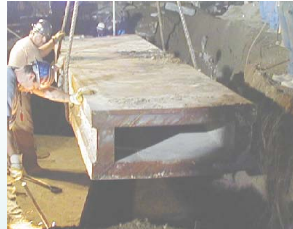
Core box column
