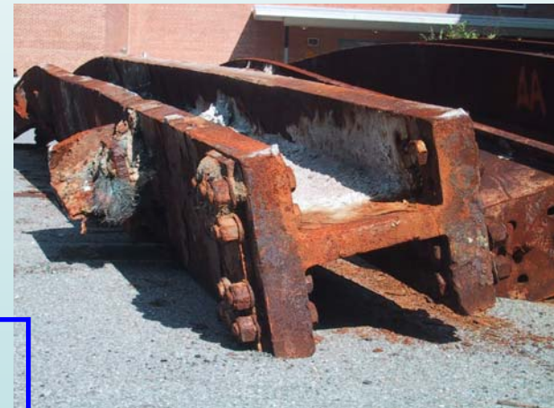
Core wide flange (WF) column
