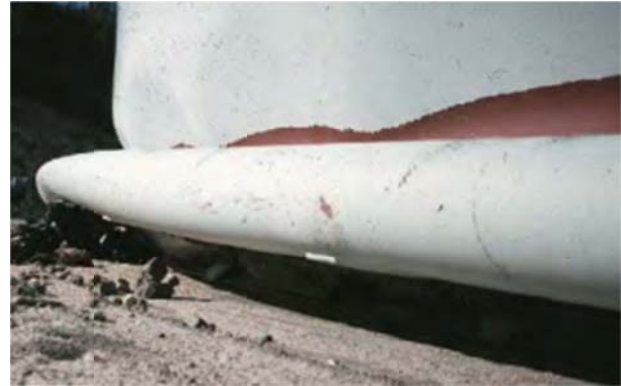
Figure 9-11: Steel Tank "Elephant's Foot" Buckling, Northridge Earthquake, California, 1994 (Source: Photo by Don Ballantyne)
