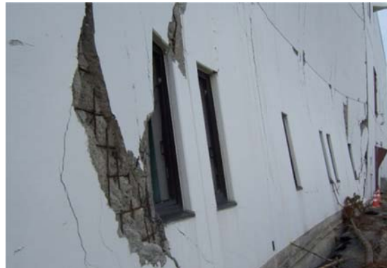
Figure 9-30: Structural Damage From Tsunami Wave and Debris Impact, Tohoku Earthquake, Japan, 2011 (Source: Tang & Edwards, 2014)
