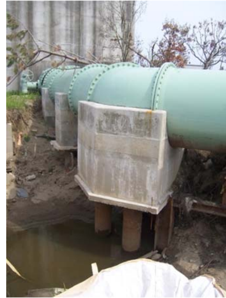
Figure 9-27: Eroded Pipe Support Foundation due to Tsunami Scour, Tohoku Earthquake, Japan, 2011 (Source: Tang & Edwards, 2014)
