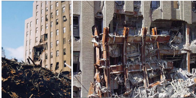
Figure 8-2. Damage to Verizon Building on September 11, 2001 (FEMA 2002)
