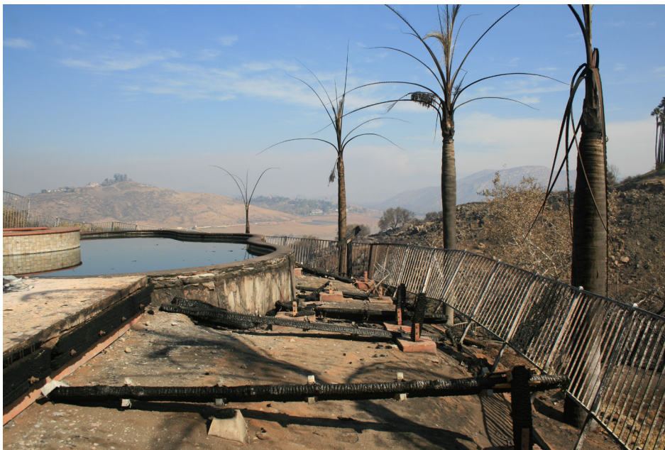
Fig. 1 Wood decking assembly ignited in the Guejito/Witch fire in Rancho Bernardo, CA. The ignition of the deck resulted in the loss of the structure.
