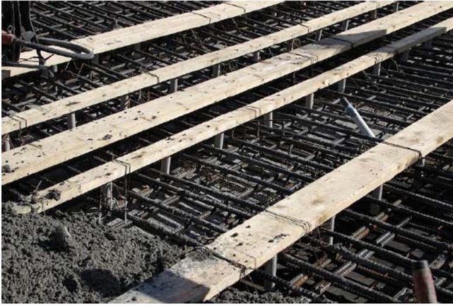
Fig. 3. A railway bridge deck with dowels and wooden planks installed.
