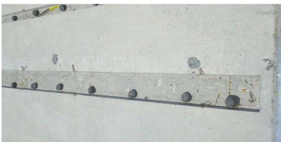
Fig. 4. Embedment holes with block-outs removed and foam plugs inserted.
