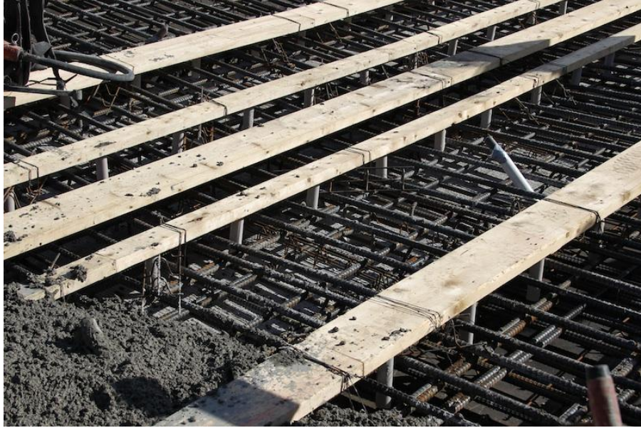
Figure 3-2 A picture of the railway bridge deck with the dowels and wooden planks installed.
