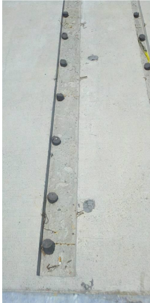
Figure 3-3 Embedment holes with blockouts removed and foam plugs inserted.
