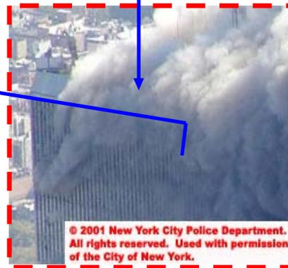
Figure 7–3. Impact damage to north and west faces of WTC 1.
