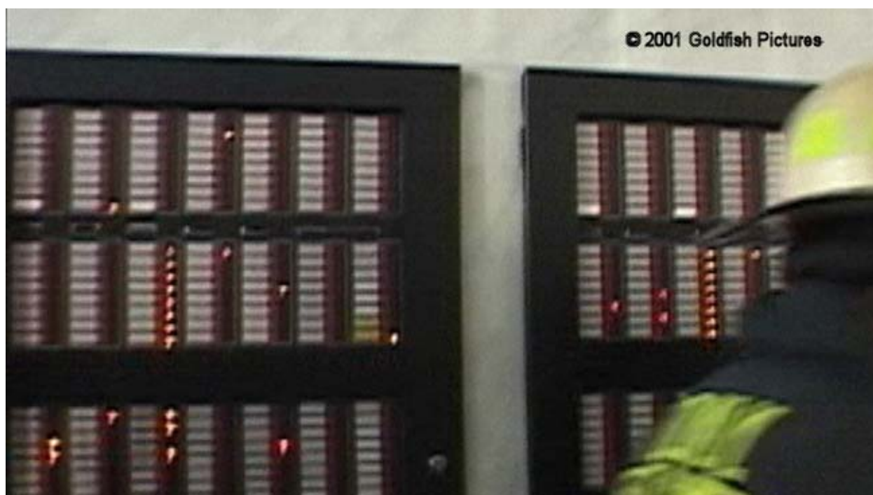
Figure 6–1. WTC 2 speaker and telephone circuit faults.
