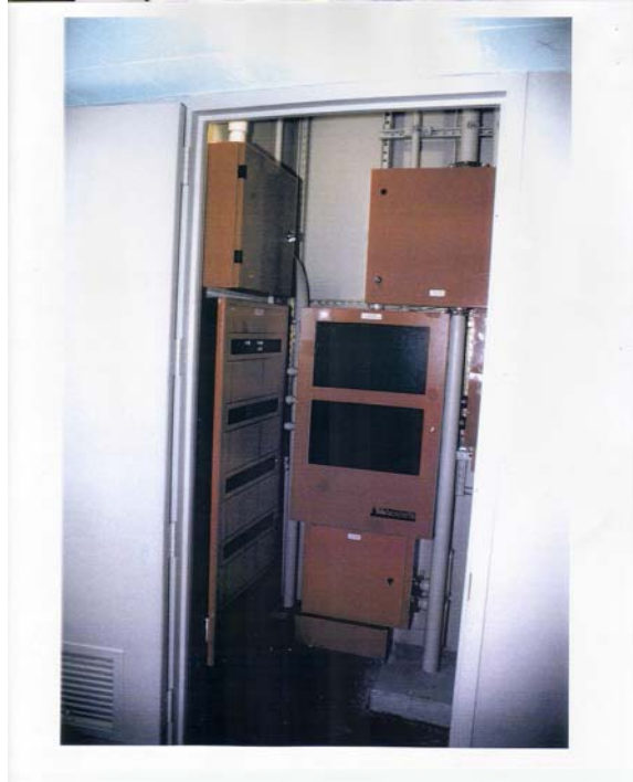
Figure 5–19. Fire alarm closet with PSR location.
