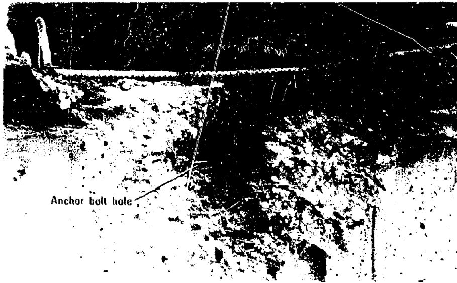
Figure 3.11 Close-up View of Top of Lift 27 Showing an Anchor Bolt Hole in Concrete
