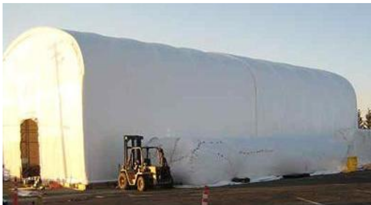
Figure 4 – Decontamination containment tent surrounds the building
