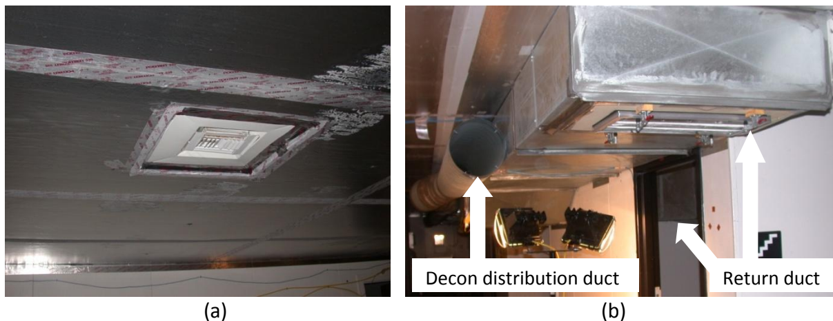
Figure 5 – (a) Rigid, foil-faced insulation attached to ceilings and (b) Retrofitted decontamination and return air ducts
