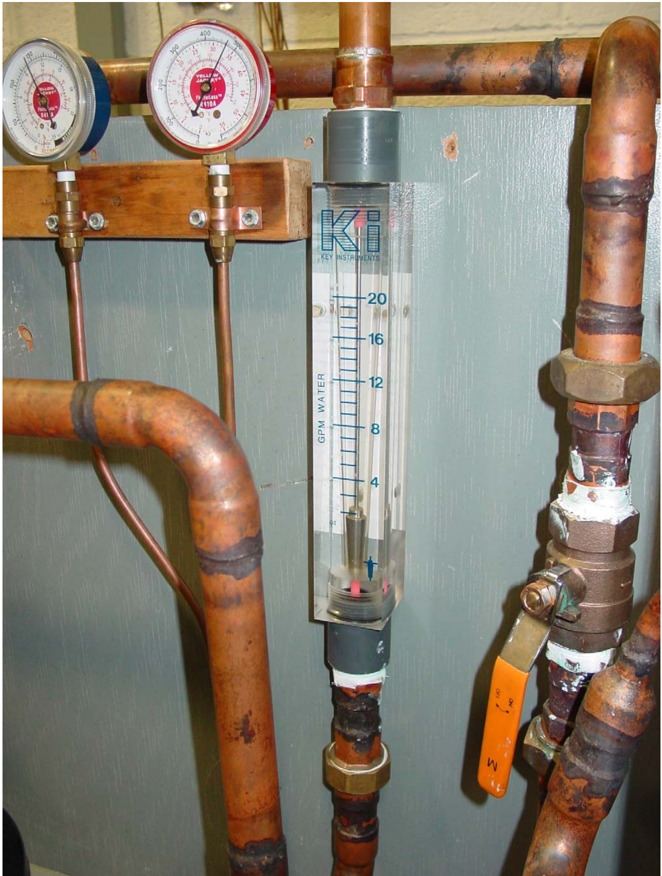
Figure B3: Rotameter/flowmeter used to adjust water flowrate to condenser heat exchanger
