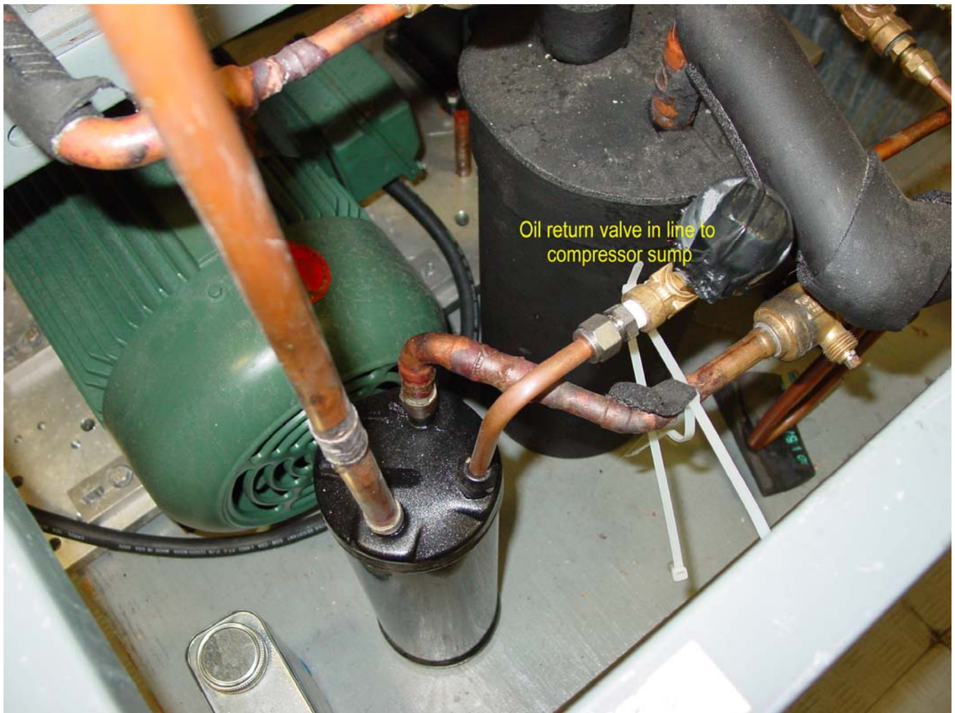
Figure B2: Oil separator arrangement
