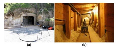
**Fig. 9.2** (a) Portal into the Hazel-Atlas mine tunnel. (b) Wood shoring approximately 150 m into the tunnel. The robot tested can be seen on the cart between the railroad tracks
