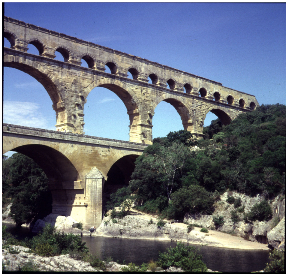
Fig. 1. Pont Du Gard, a bridge and aqueduct constructed by the Romans. The aqueduct is lined with cement composed of slaked lime and volcanic scoria [1].
