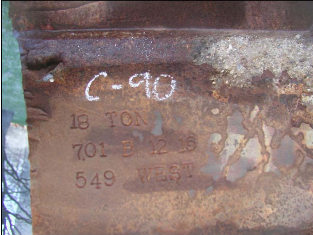
Figure 5–2. Example of stampings placed on one end of a core column. Shown here on sample C-90 are the stampings “18 TON, 701 B 12 – 16, 549 WEST,” indicating that it is from WTC 2, core column number 701, and spans floors 12 to 16. Also indicated are the approximate weight of the piece (18 tons) and the derrick division <549> that was to lift it into place.
