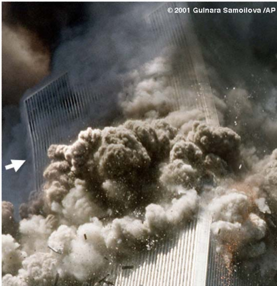
Figure 6–19. Initial seconds of collapse of WTC 2 viewed from the east-northeast, and kink in the southeast edge of the building near the 106th floor (arrow).
